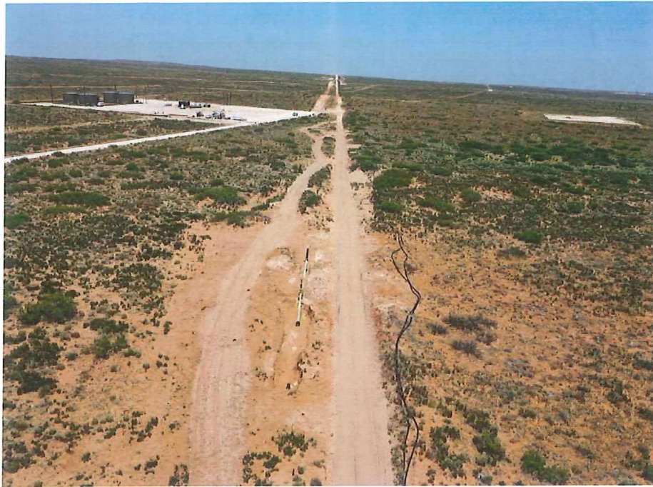
Aerial View Backfilled Excavation, Drone Image
