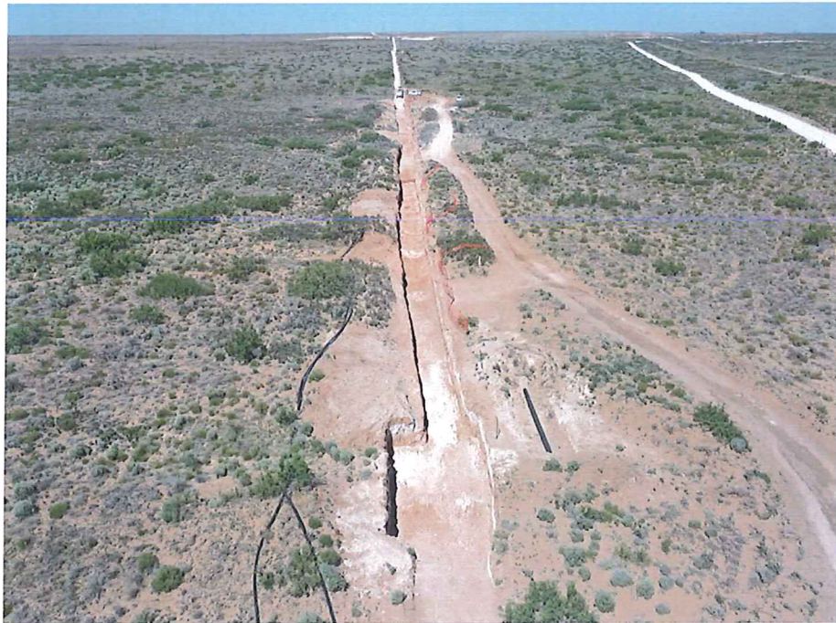
Aerial View Excavation, Drone Image
