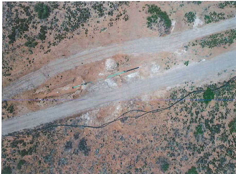
Aerial View Backfilled Excavation, Drone Image
