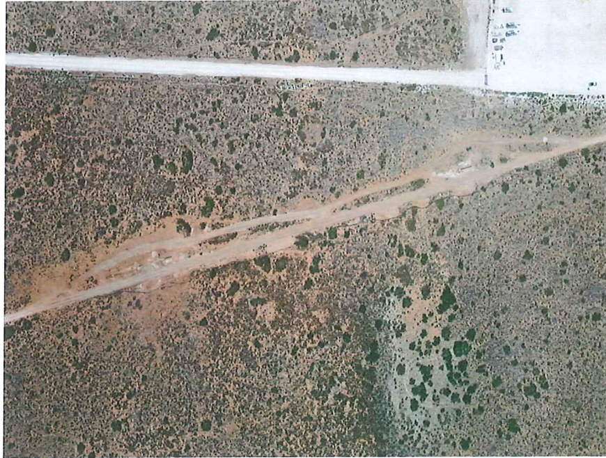
Aerial View Backfilled Excavation, Drone Image
