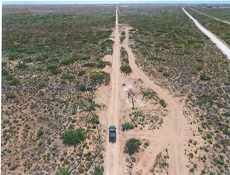
Aerial View Backfilled Excavation, Drone Image
