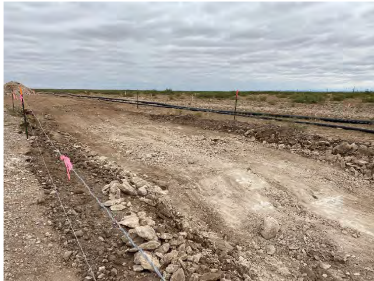
Photograph 3: Southern view of September 11 th excavation down to caliche.
