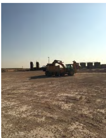
29. View of backhoe dumping contaminated dirt into dump truck to be disposed of.
