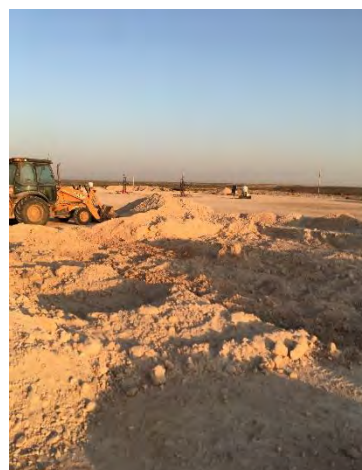
28. View of excavation of SS-11 with contaminated soil and backhoe visible.
