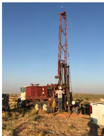
18. View of installation of MW-1 to monitor depth to groundwater.
