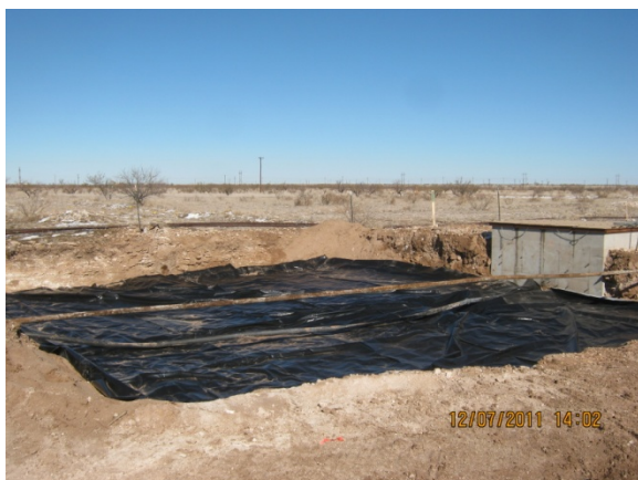
20-mil reinforced plastic liner installed at 4.5 ft BGS, facing northeast 12.7.11
