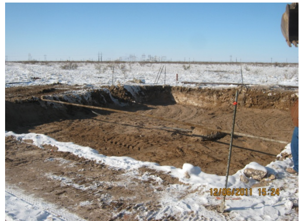
Installed bottom 6" sand pad, facing northwest 12.6.11
