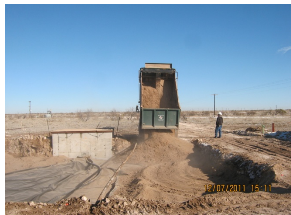
Installing 6" sand pad above liner with imported blow sand, facing east 12.7.11
