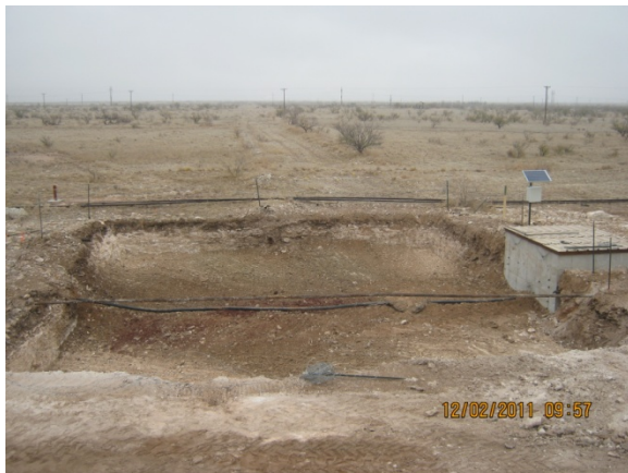
Site excavated to 49x44x5-ft deep, facing north 12.2.11
