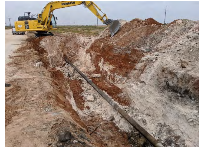
Initial Excavation Looking West (9/11/20)
