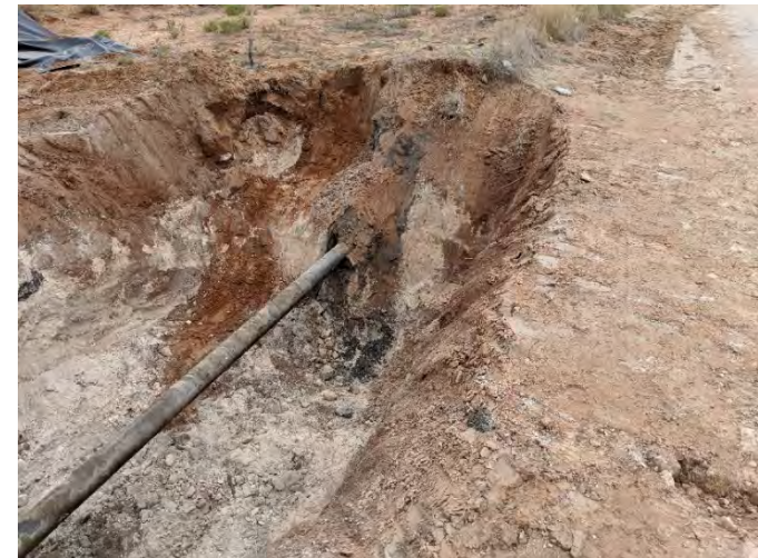
Initial Excavation Looking East (9/11/20)
