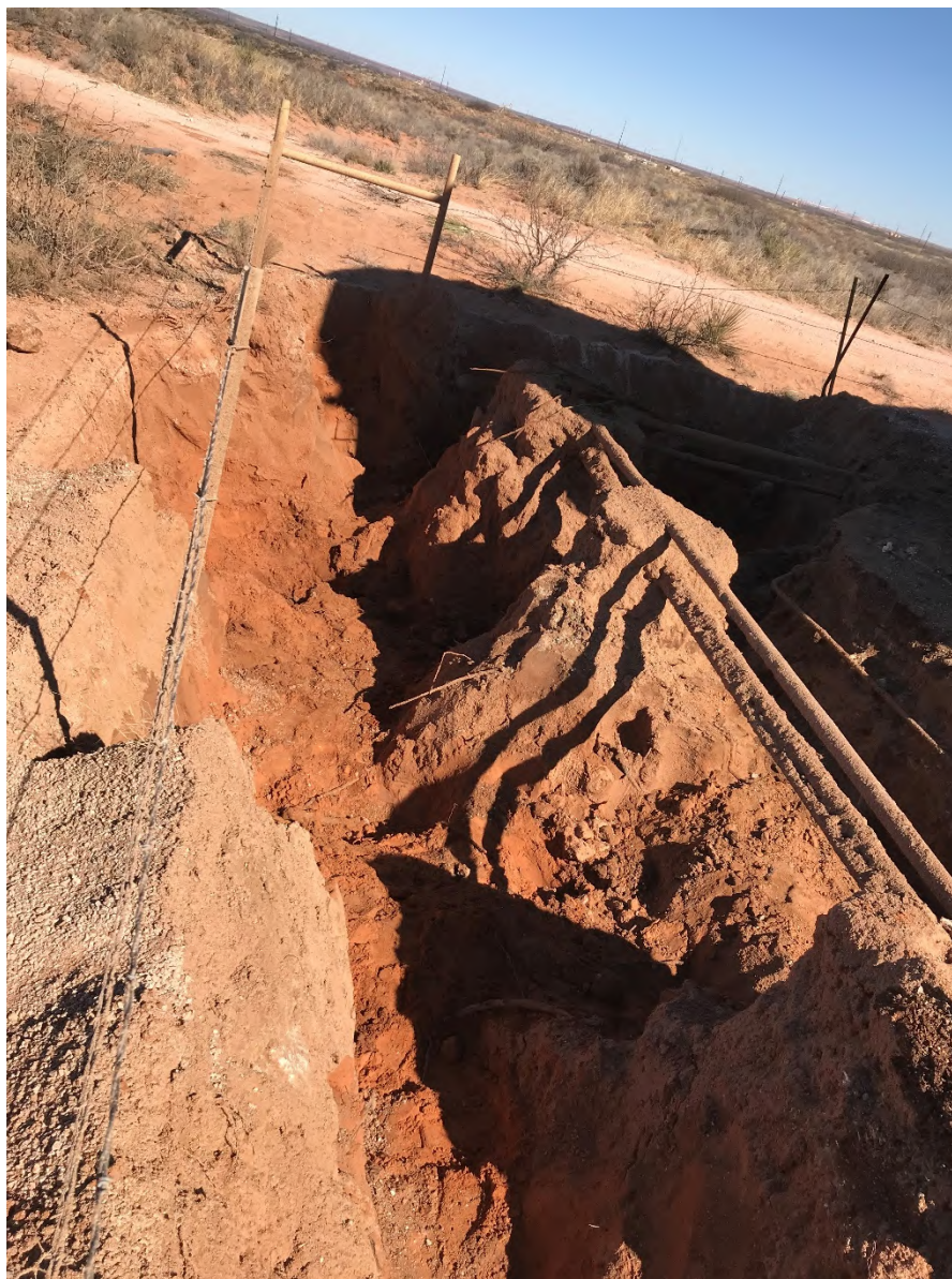
View facing west of initial excavation activities.
