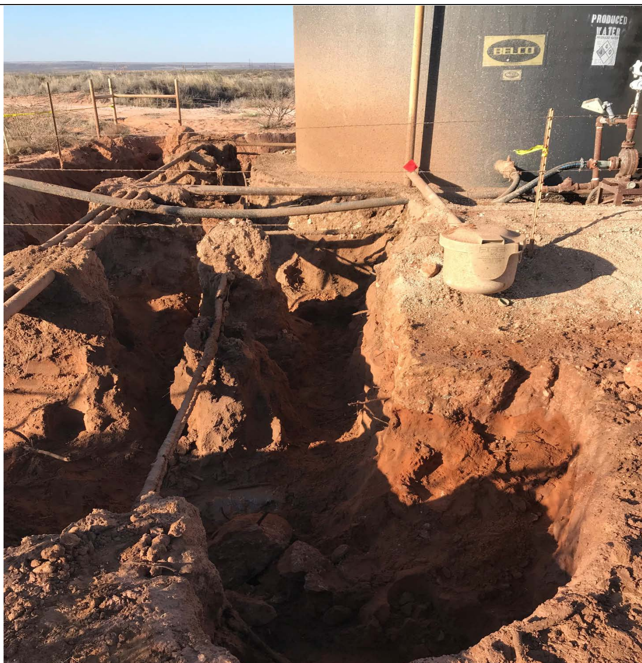
View facing north of initial excavation activities.
