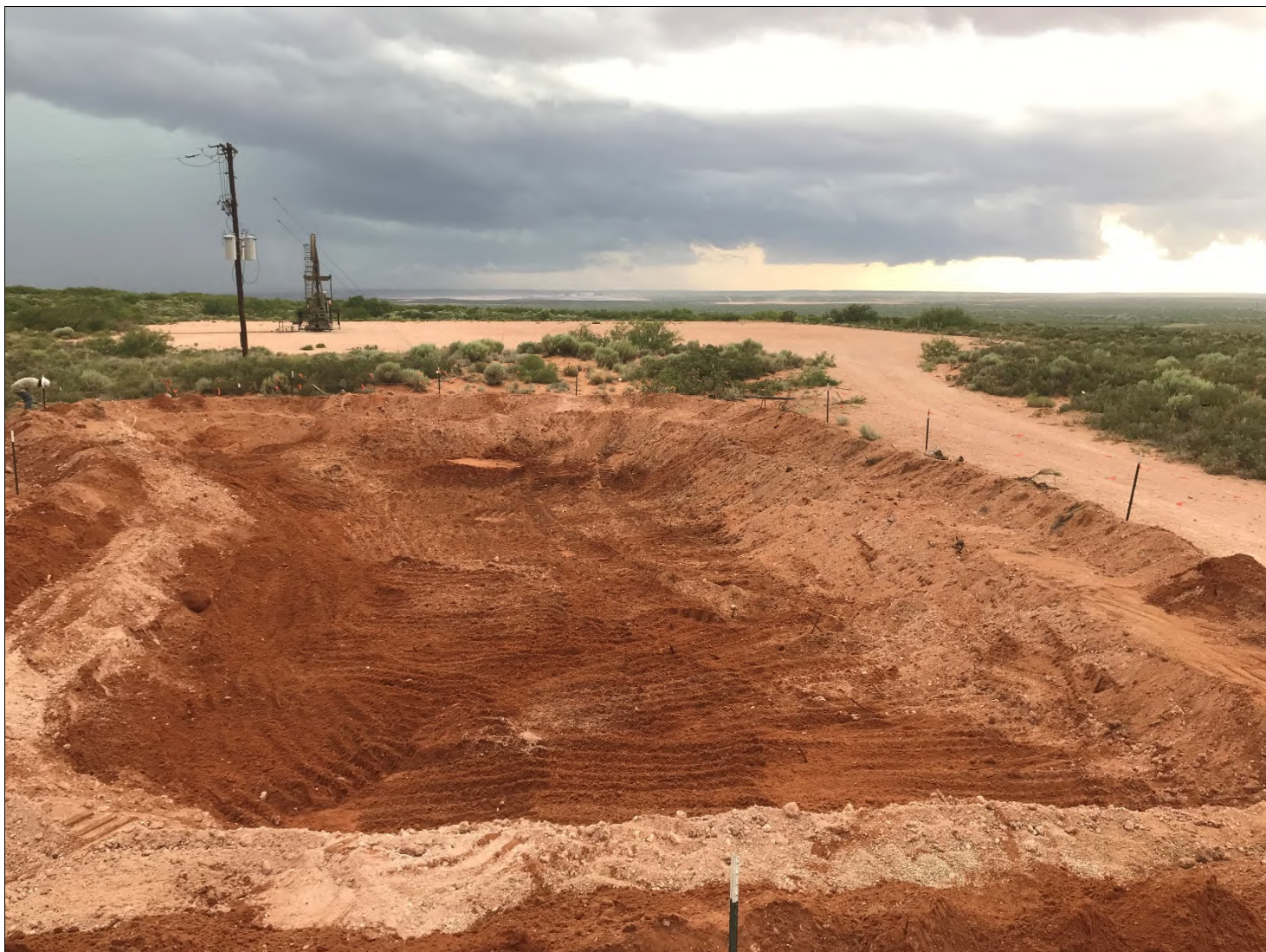
View facing west post tank battery removal.
