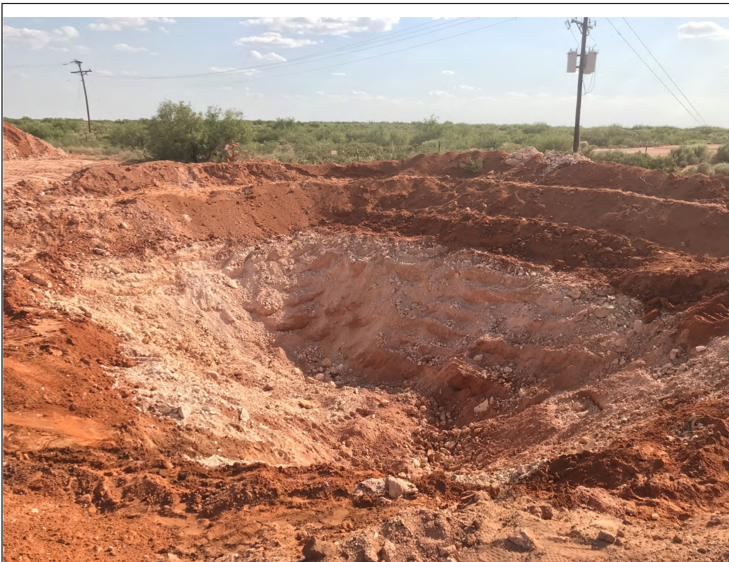
View facing southwest of the open excavation.
