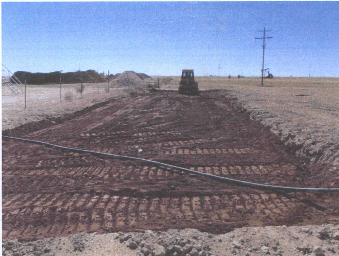
Photograph (looking West) of Clay Cap installation at the LR Chamberlain Tank Battery.
