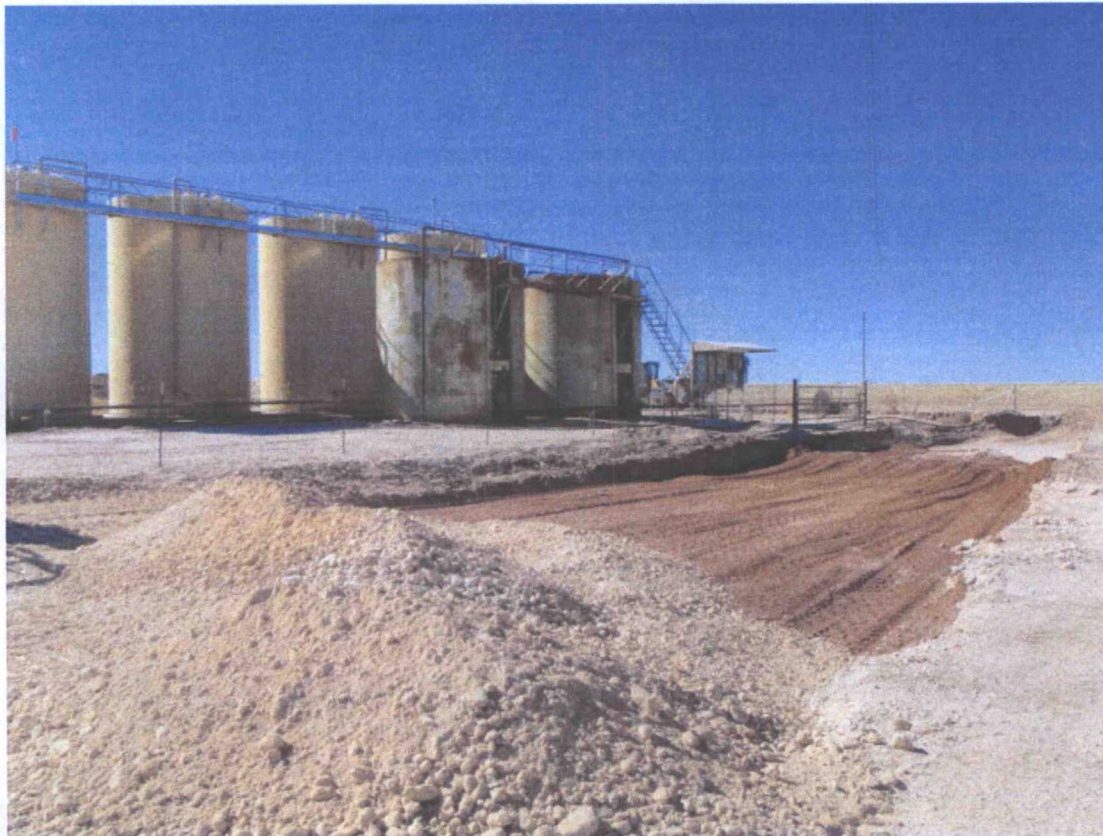
Photograph (looking Southeast) of Caliche being installed over Clay Cap at the LR Chamberlain Tank Battery.
