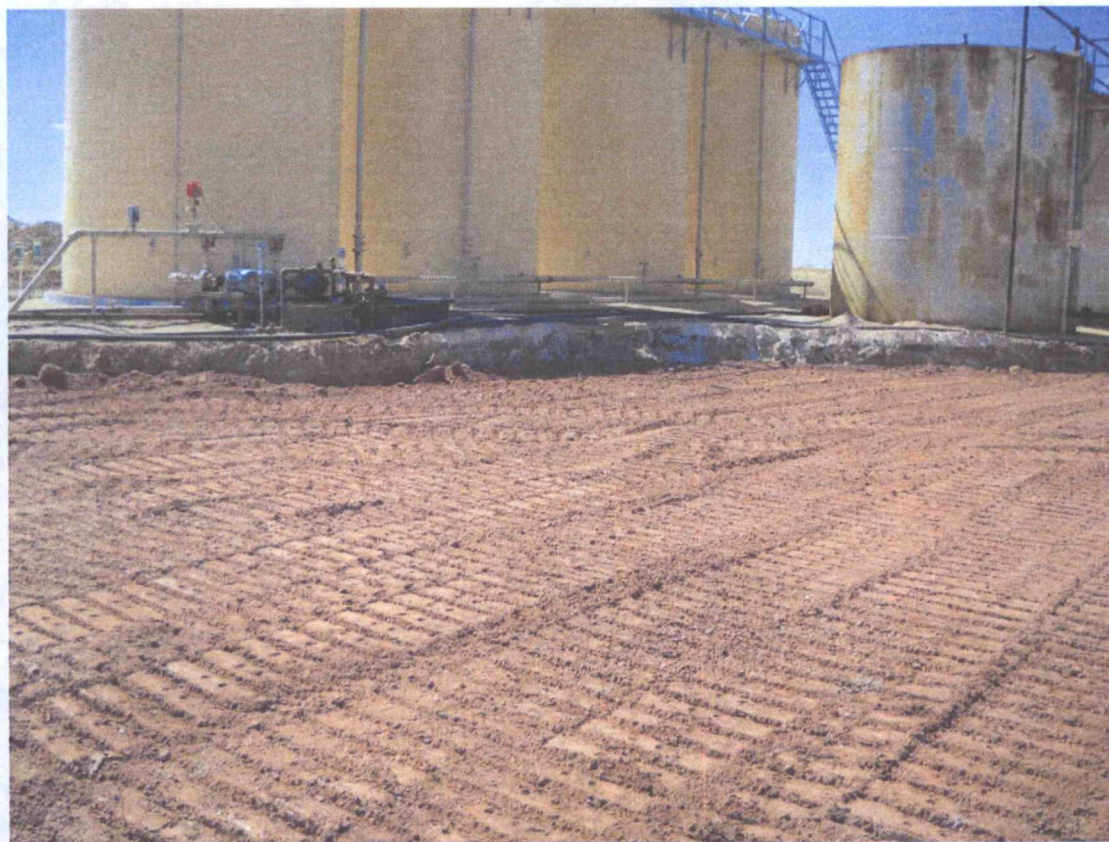
Photograph (looking Southeast) of the Clay Cap at the LR Chamberlain Tank Battery.
