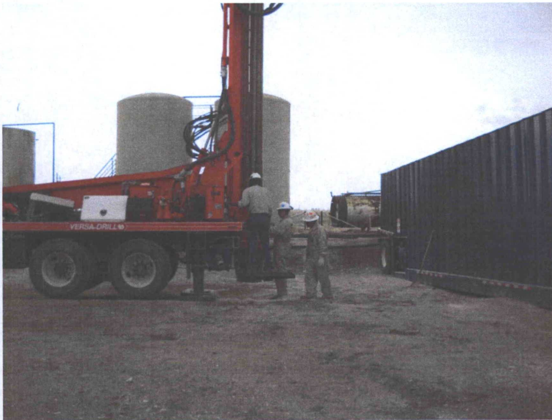
Photograph (looking North) of advancement of Soil Boring SB-1 at the LR Chamberlain Tank Battery.
