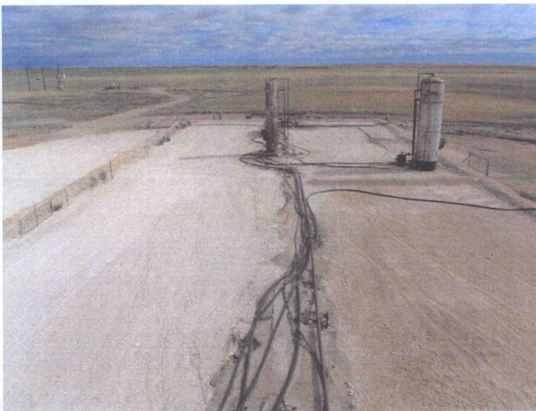
Photograph (looking East) of the newly installed caliche and completed remediation activities at the LR Chamberlain Tank Battery.
