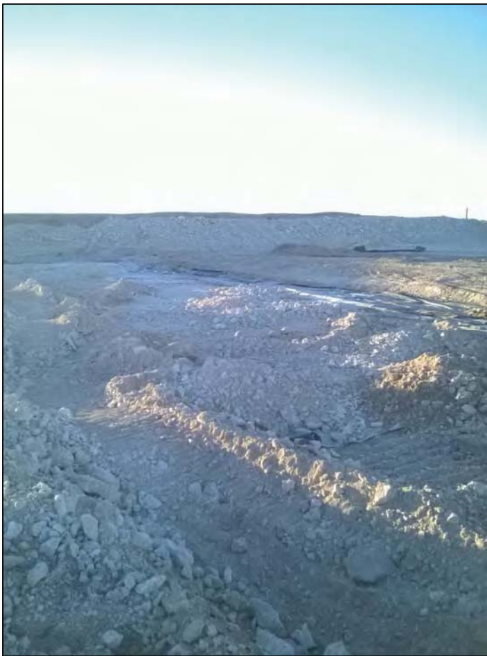
Backfilling over geomembrane cover 12/30/2014
