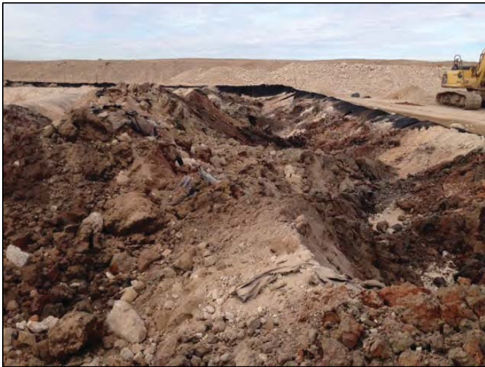
Mixing pit contents with trackhoe 12/3/2014
