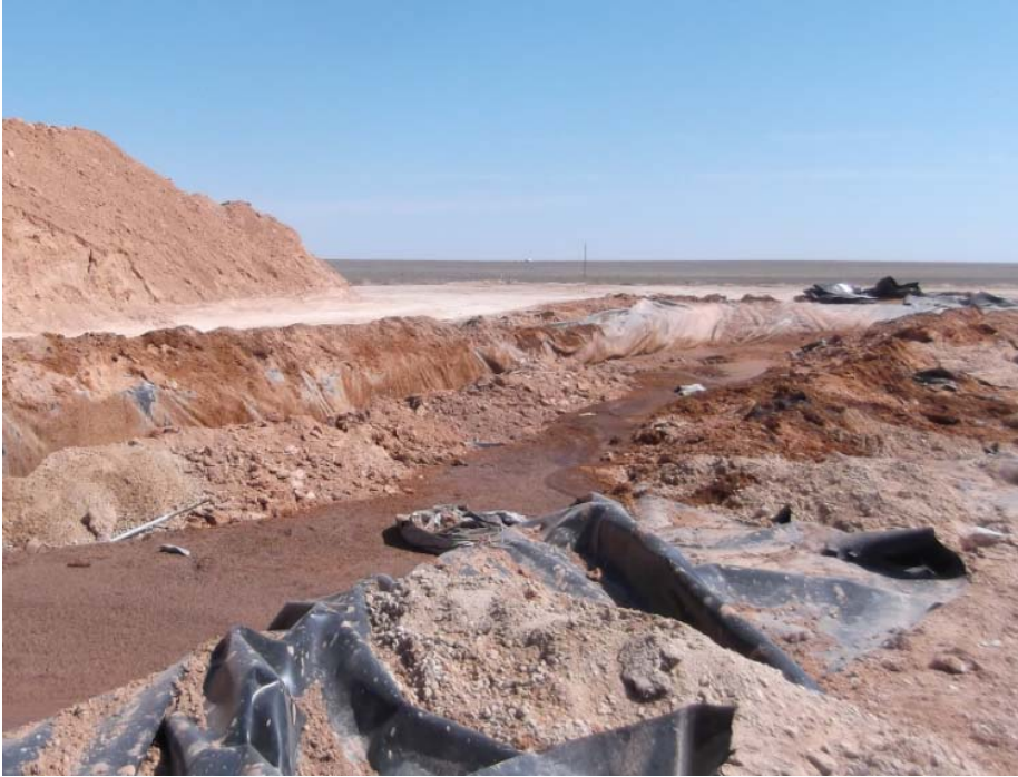
Figure 2: View to northeast during placement of stabilized material from the temporary pit into the burial trench. The material was later shaped to have a slightly domed top before placement of the upper liner
