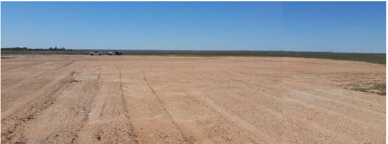
Figure 3: View to south and southwest of completed top soil surface from the northern side of the burial trench (Photo taken on April 2, 2015). The topography was sloped to be higher over the burial trench and slopes down to the location of the former temporary drilling pit, in the left and center middle ground. Soil from the original excavation had been stockpiled on the right middle ground.
