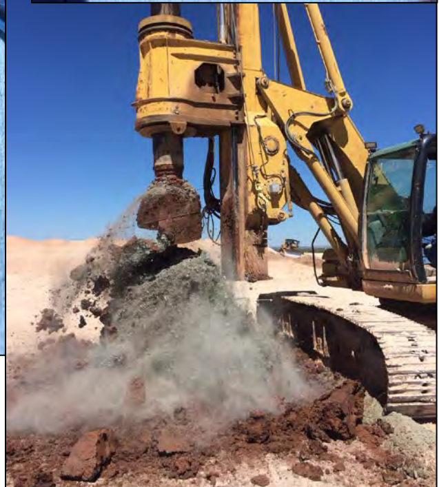
Final TOOH: Dry, gray clay at 80 ft is visible at bottom half of auger
