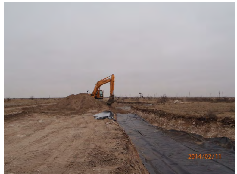
Liner installation completed and beginning backfilling the excavation, facing southeast 2/11/14
