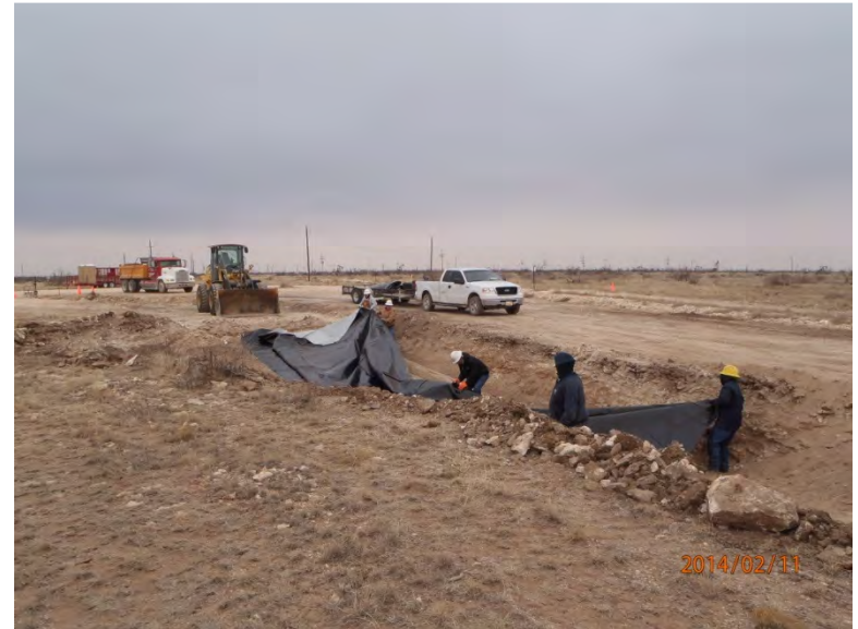
Installing 20-mil reinforced poly liner, facing north 2/11/14
