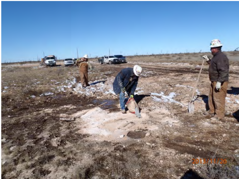
Plugging SB-1 in total with bentonite, facing northwest 11/26/13
