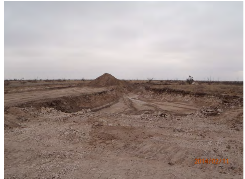
Excavation completed with the bottom padded for liner installation, facing east
