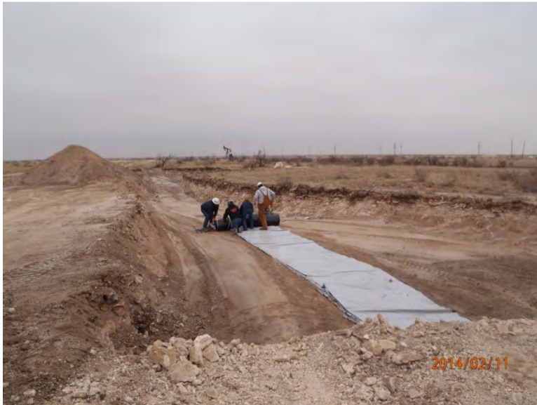
Installing 20-mil reinforced poly liner, facing southeast 2/11/14
