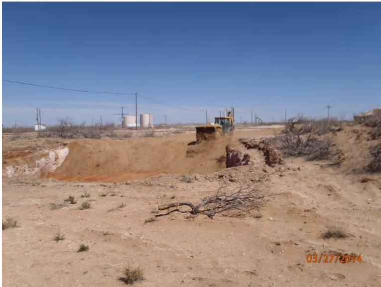
Backfilling east excavation with top soil, facing north 3/27/14
