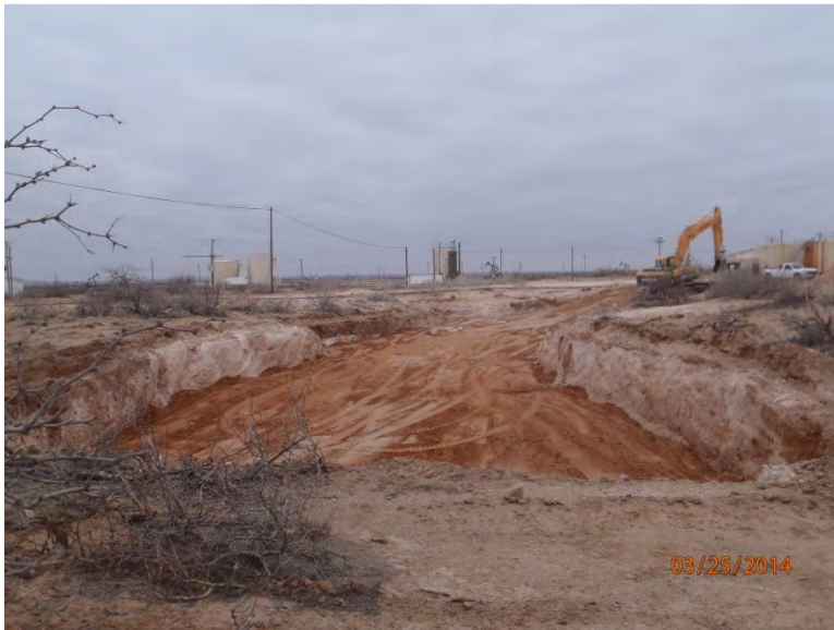
Clay liner installed in east excavation, facing north 3/25/14
