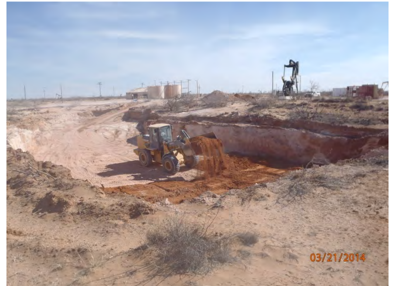
Installing clay liner in east excavation, facing northeast 3/21/14
