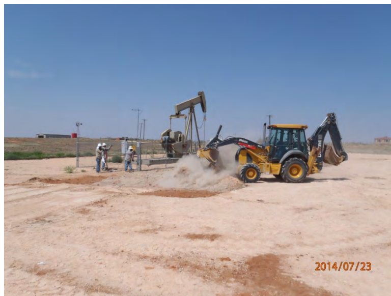
Backfilling with imported caliche, facing southwest 7/23/14
