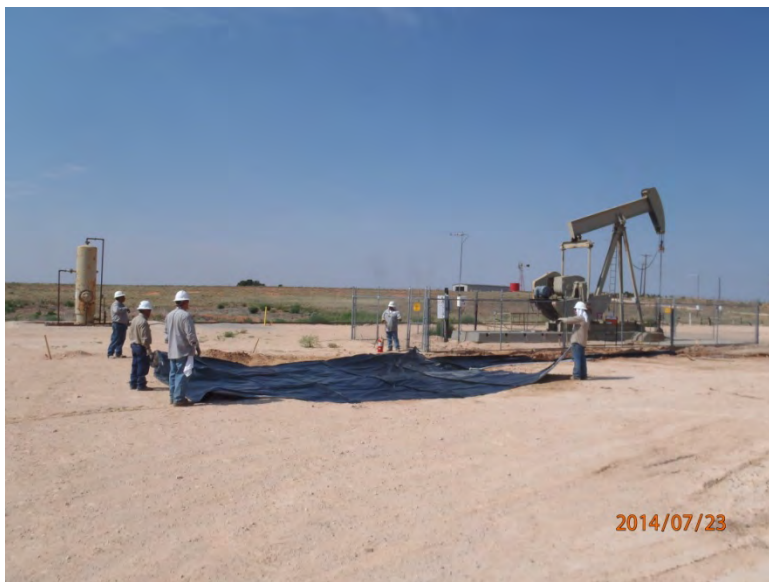
Installing 20-mil reinforced poly liner at 1.5 ft, facing south 7/23/14
