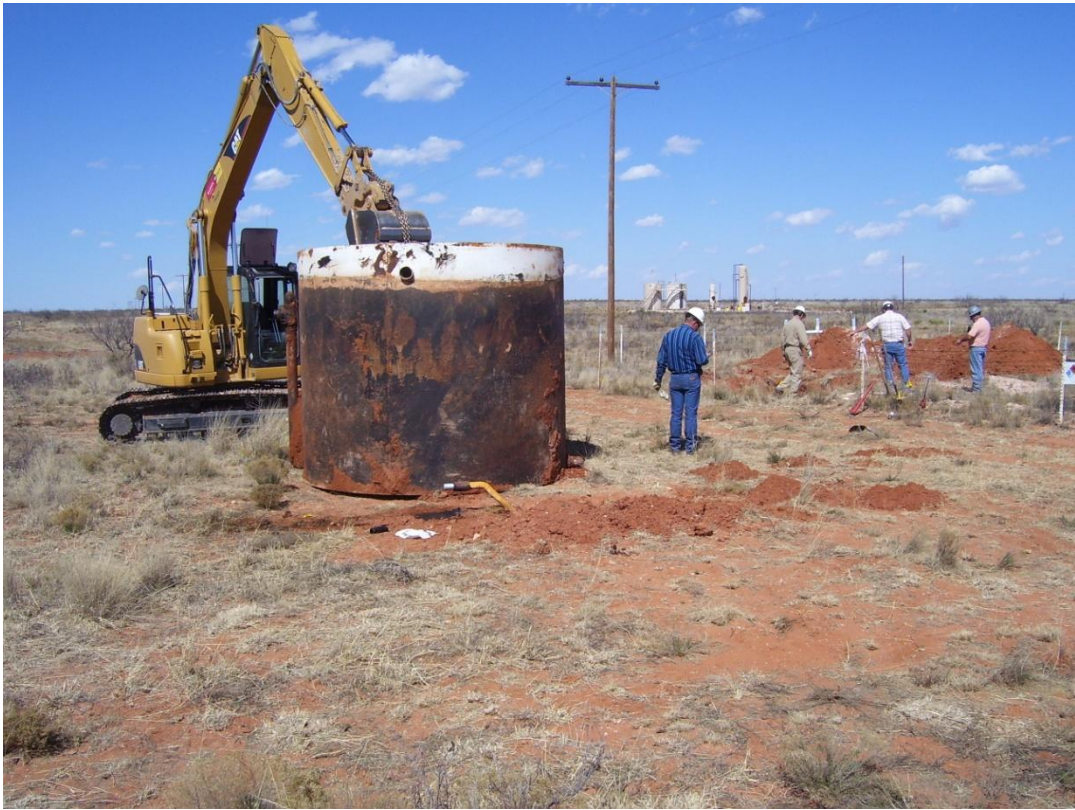
Photograph of the BGT removal at Drip Tank #106.
