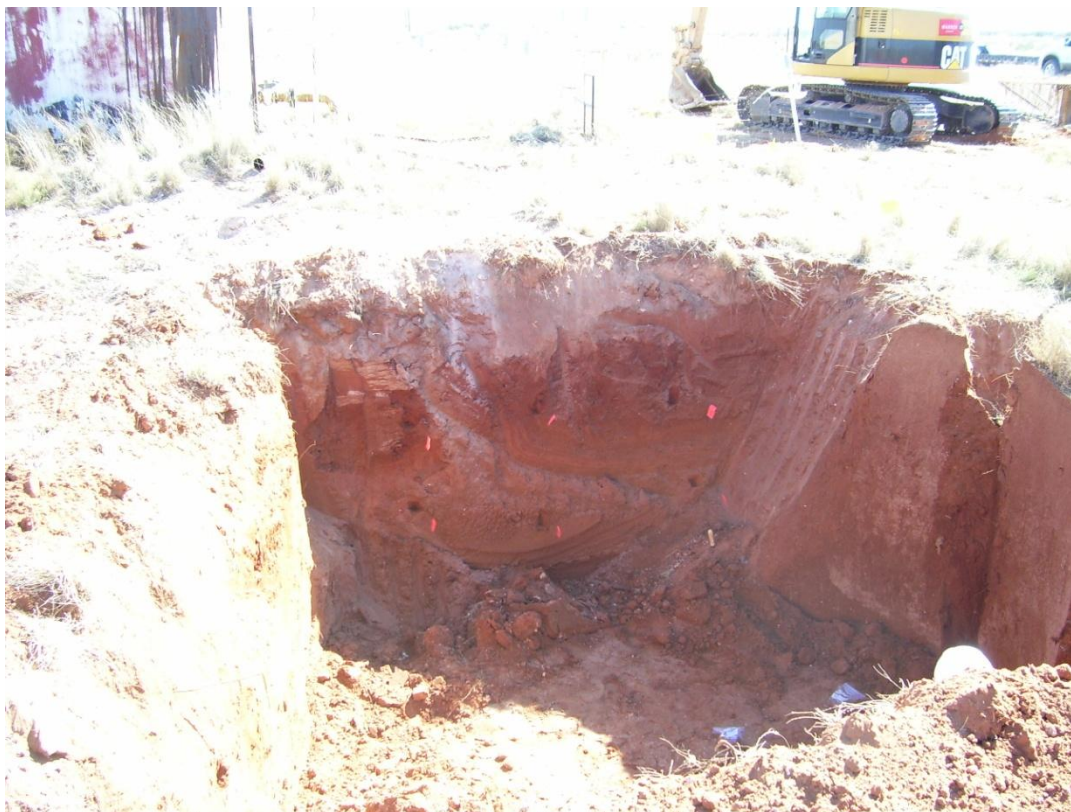
Photograph of the BGT removal and sample locations at Drip Tank #106.
