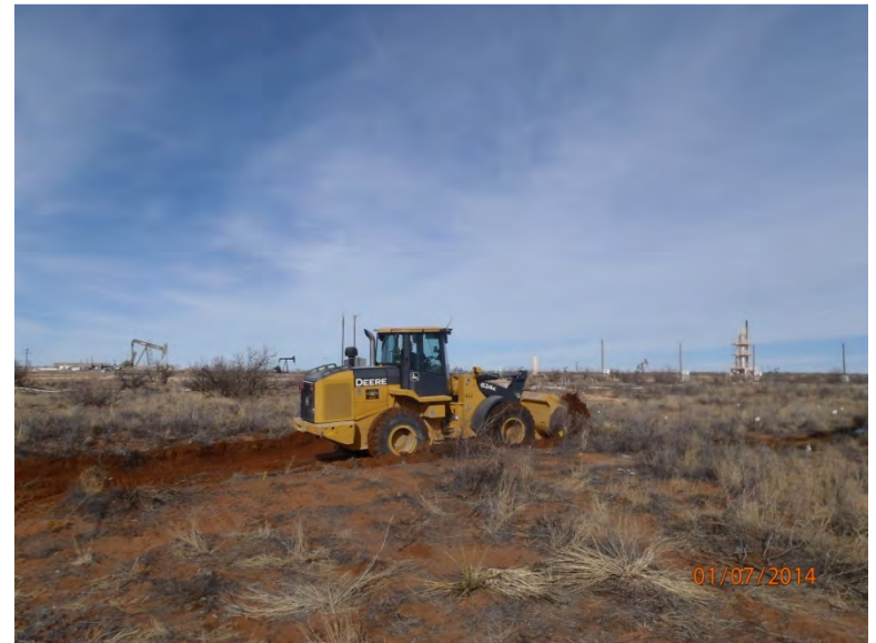
Scraping release, facing northeast 1/7/14
