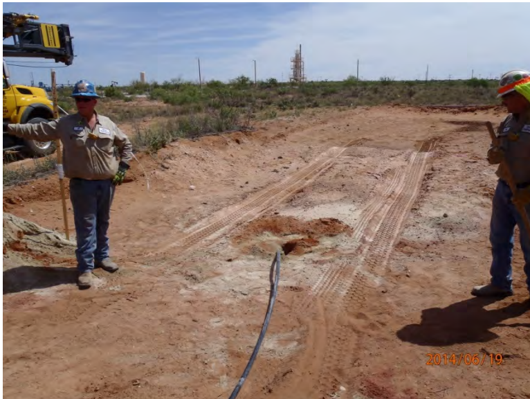
Plugging SB-2 with a cement/bentonite slurry, facing east 6/19/14
