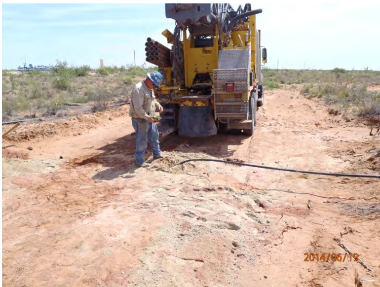
Plugging SB-3 with a cement/bentonite slurry, facing northeast 6/19/14
