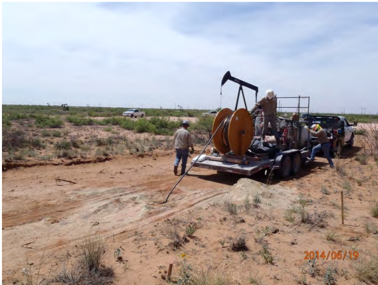
Plugging SB-1 with a cement/bentonite slurry, facing southeast 6/19/14
