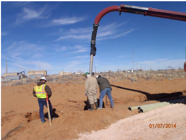
Hydro-excavating, facing northeast
