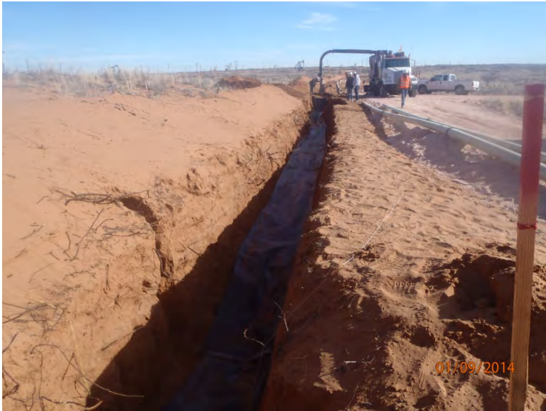
Installed liner, facing east
