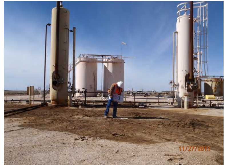
Plugging augur point in total with bentonite, facing west
