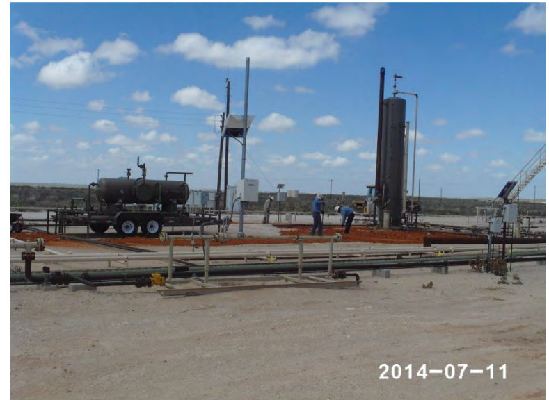
Backfilling site with clay, facing southwest
