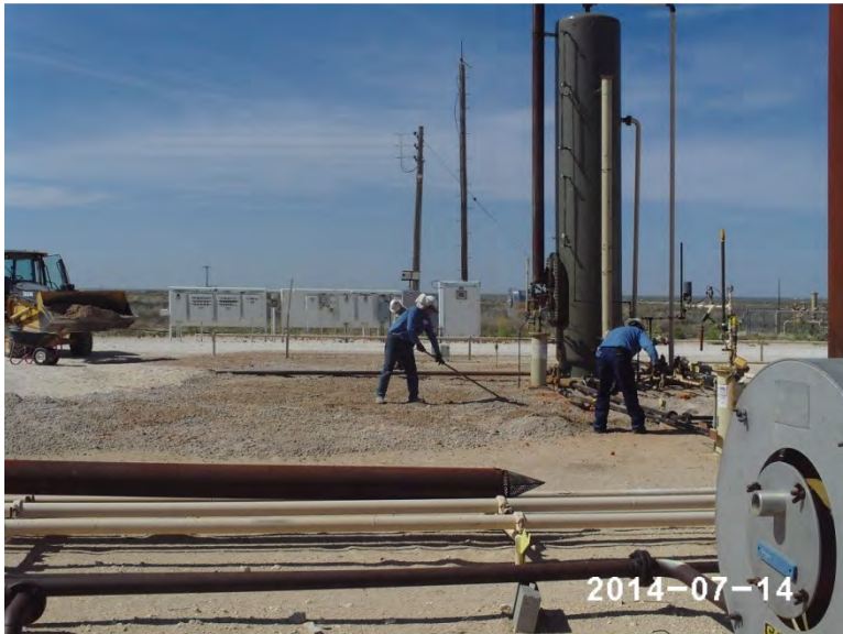
Backfilling the site with caliche, facing south 7/14/14
