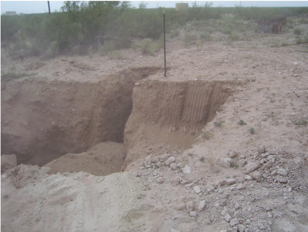
Photograph of excavation and delineation trenches advanced during initial investigation at the Trunk "O" Tank Battery.
