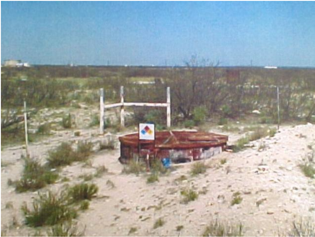
Photograph of Below Grade Tank prior to removal at the Trunk "O" Tank Battery.
