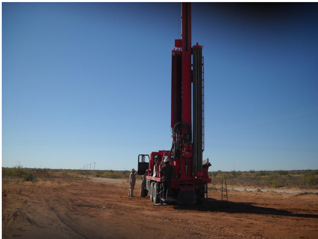
Photograph of the advancements of soil borings at the Trunk "O" Line Historical Release Site.
