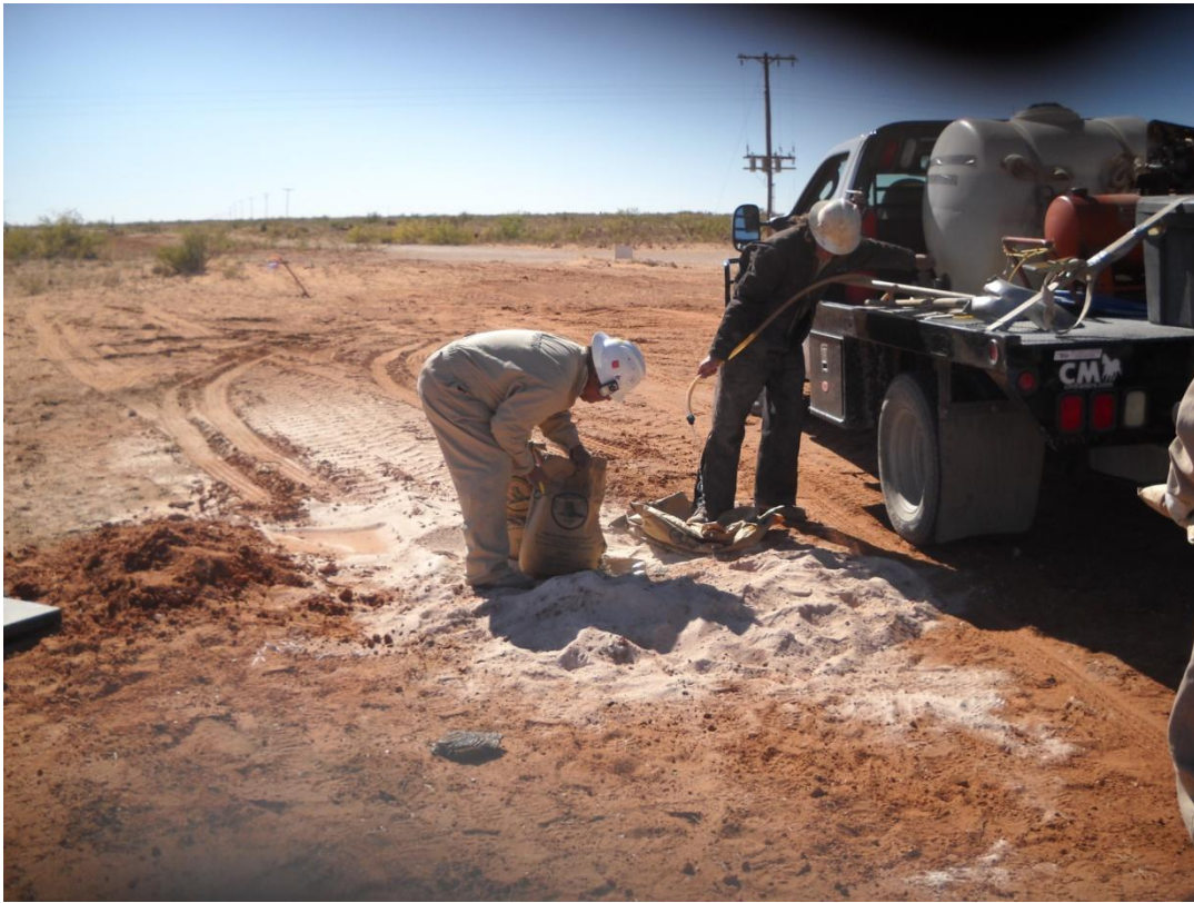
Photograph of the plugging of the soil borings at the Trunk "O" Line Historical Release Site.
