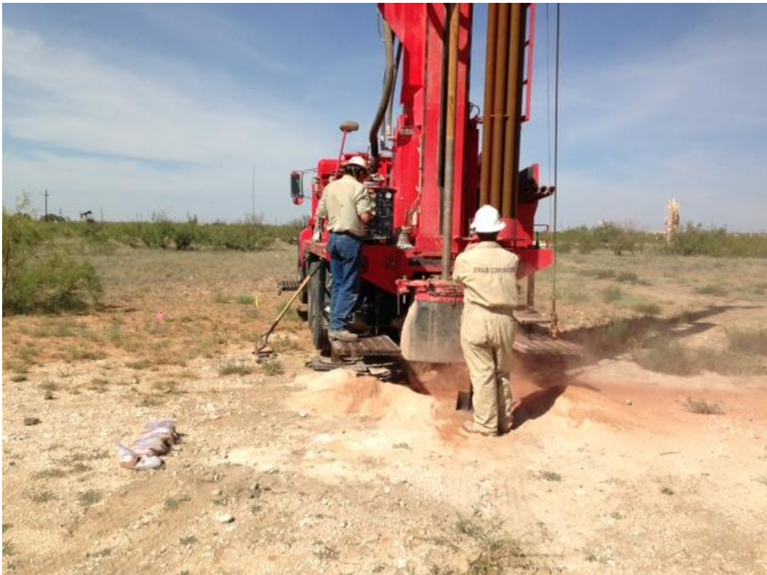
Photograph of the advancement of soil bores at the Trunk "O" #2 Historical Release Site.
