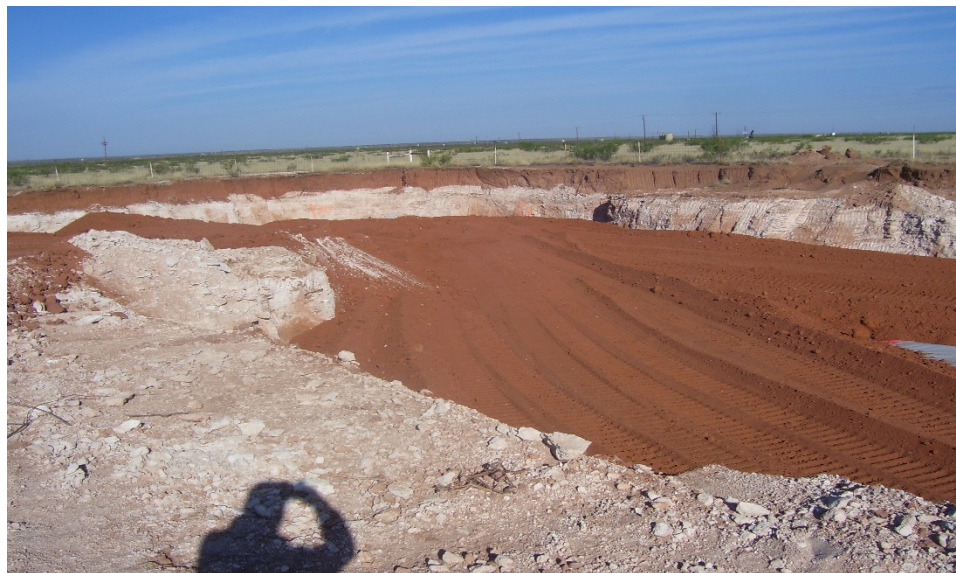
Backfill on top of Liner
