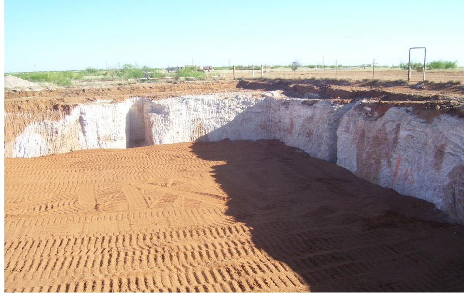
Backfill before Liner Installation
