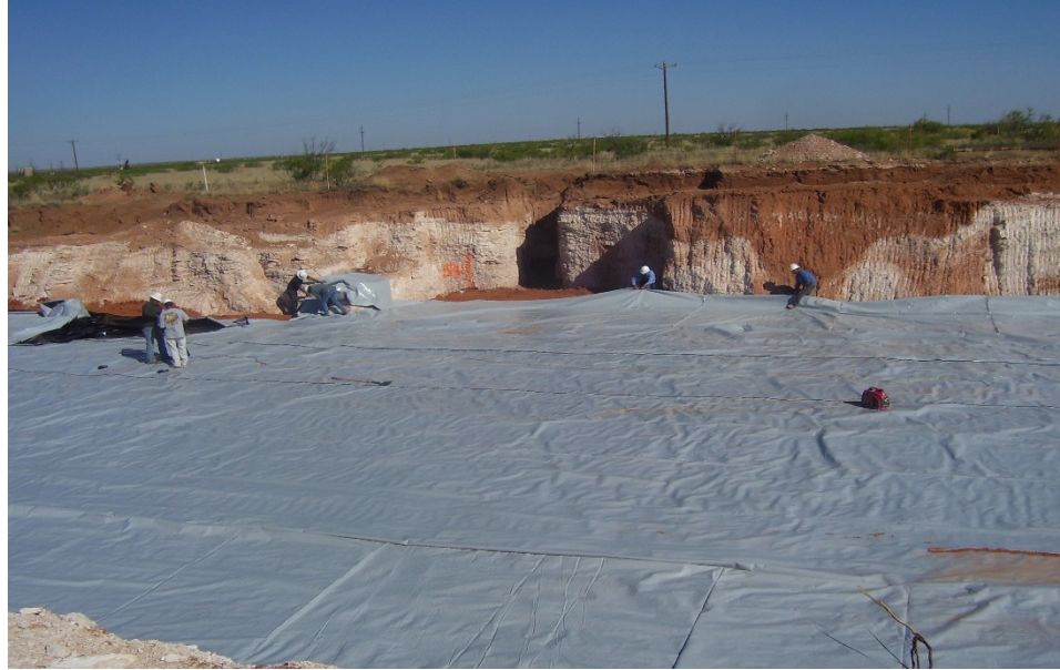
Liner Installation
