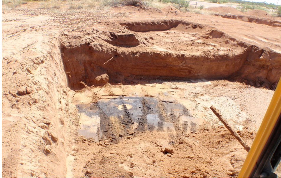
Staining from Tanks
