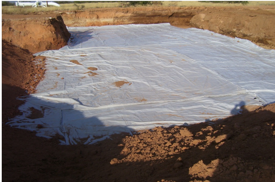
Area of Excavation, Liner Installed
