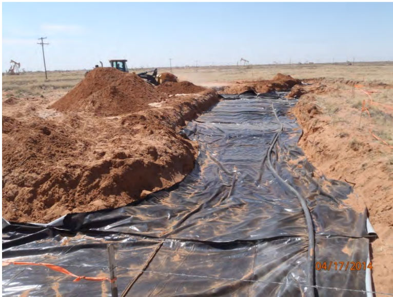
Liner installation completed, facing south 4/17/14
