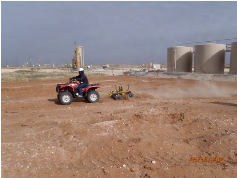
Disking soil to prepare for seeding, facing northwest 5/1/14
