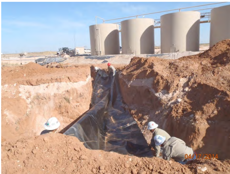
Installing liner, facing northwest
