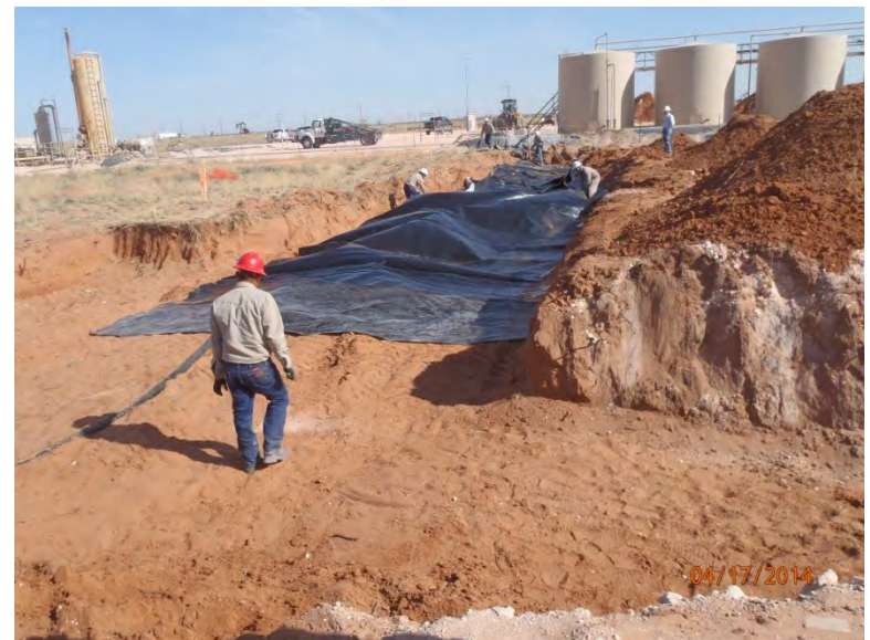
Installing liner, facing north
