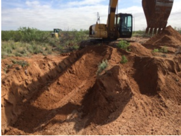
Excavating spill area to 3' bgs
