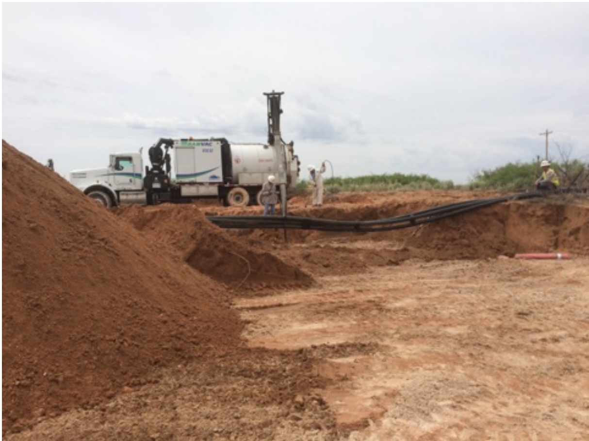
Using hydrovac to dig between trunk lines
