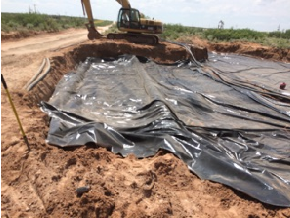
Liner installation in excavated area
