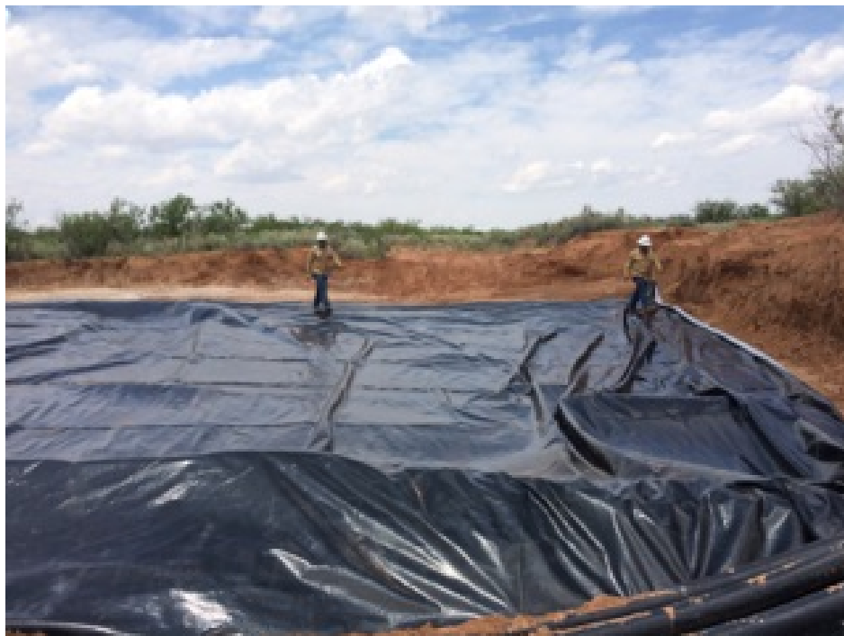
Liner installation in excavated area
