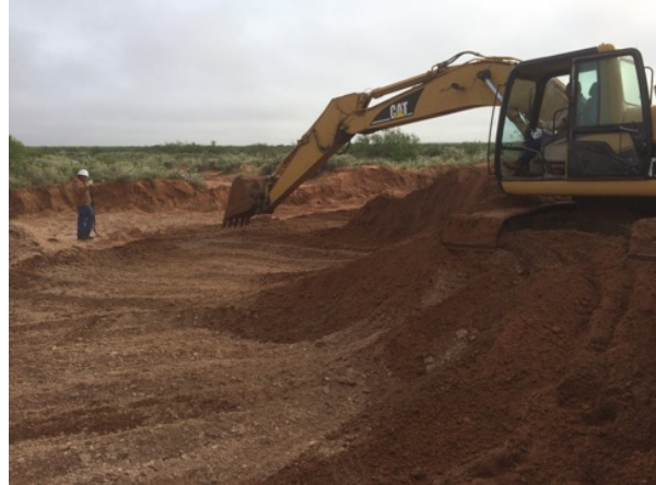
Excavating spill area to 3' bgs
