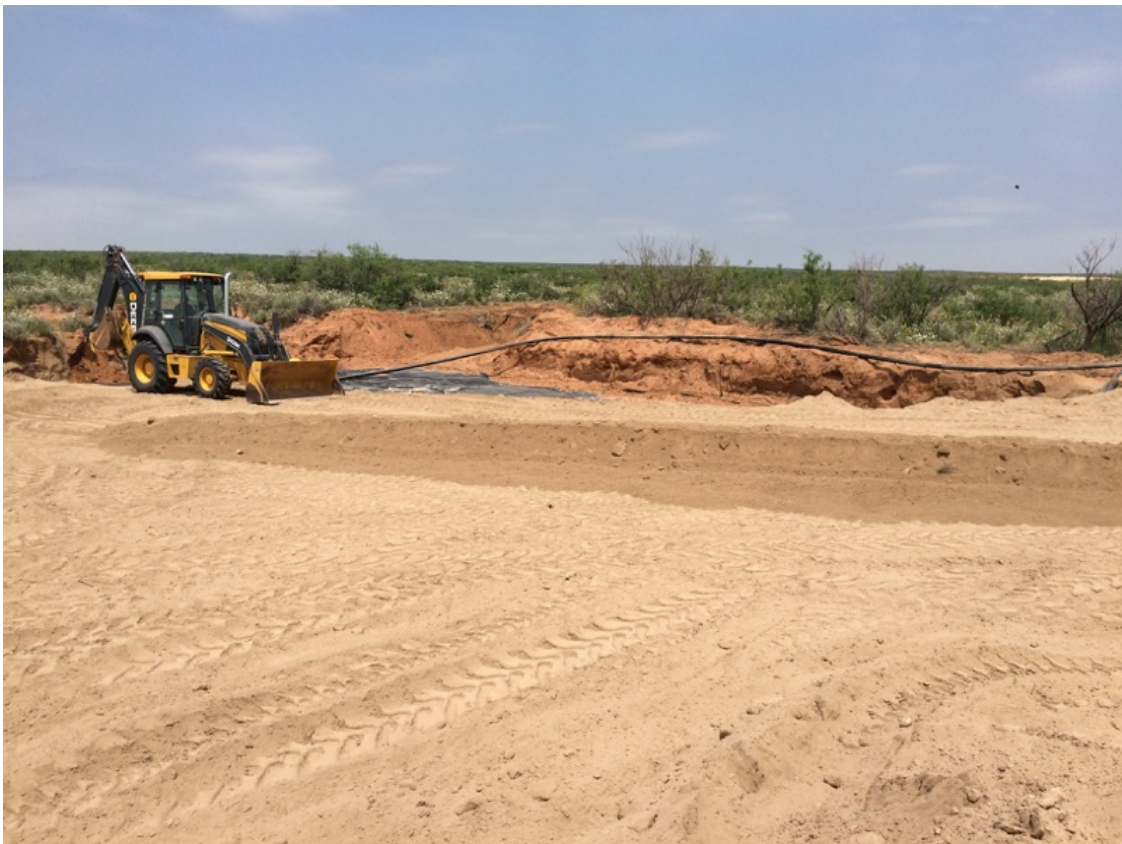
Backfilled area after liner installation
