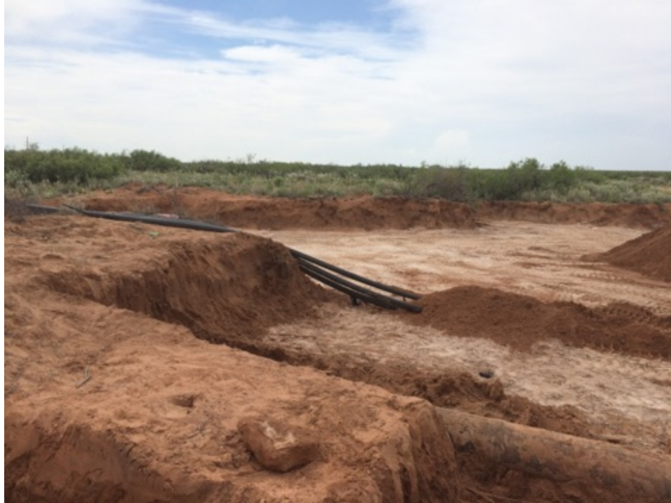
Excavated spill area, ready for liner installation
