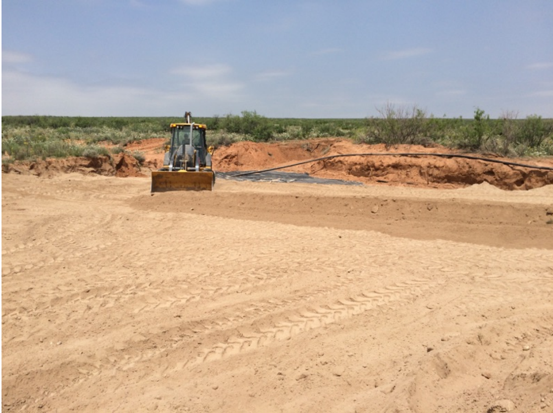
Backfilled area after liner installation
