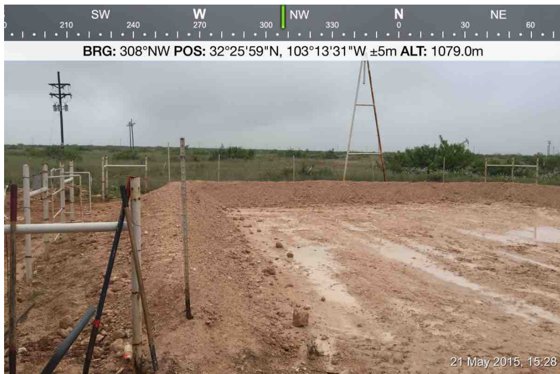
Backfilled area with fresh caliche
