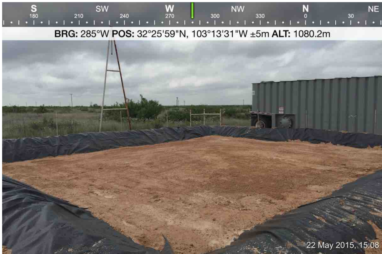
Completed location with liner installation and rebuilt berms
