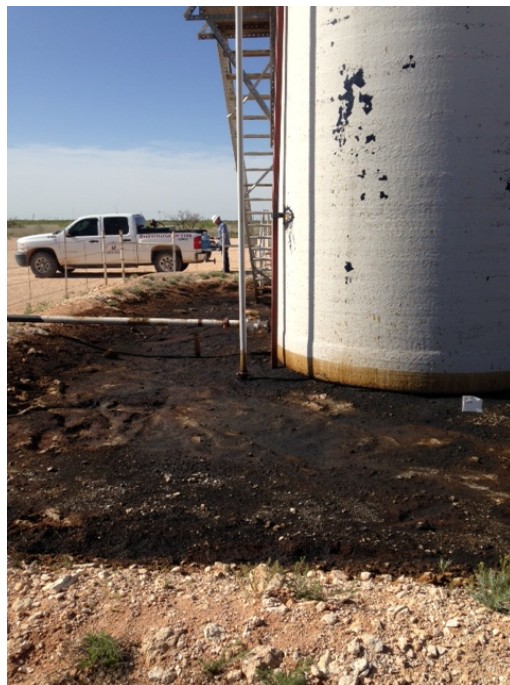
Spill area inside bermed facility
