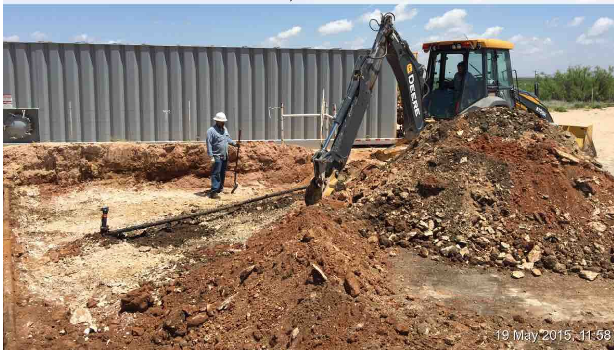
Excavating area inside bermed facility after tank removal
