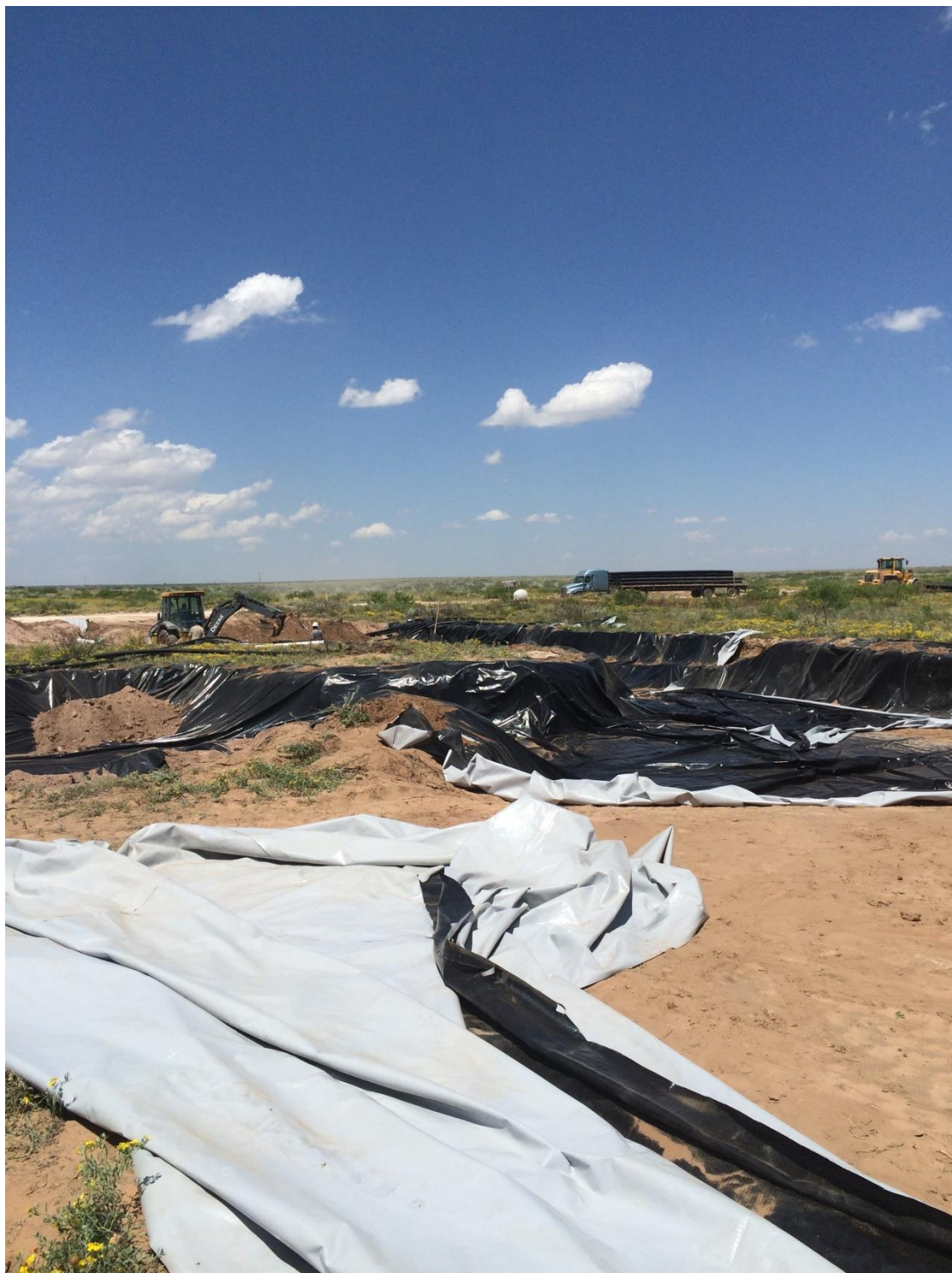
Photo 6 – Liner and backfill being placed in the excavation. Photo taken facing southeast.
