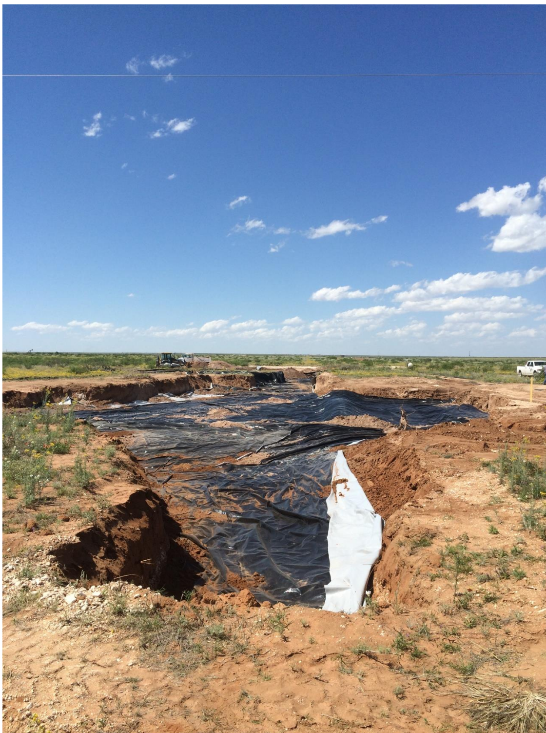
Photo 7 – Excavation after liner placement. Photo taken facing north.
