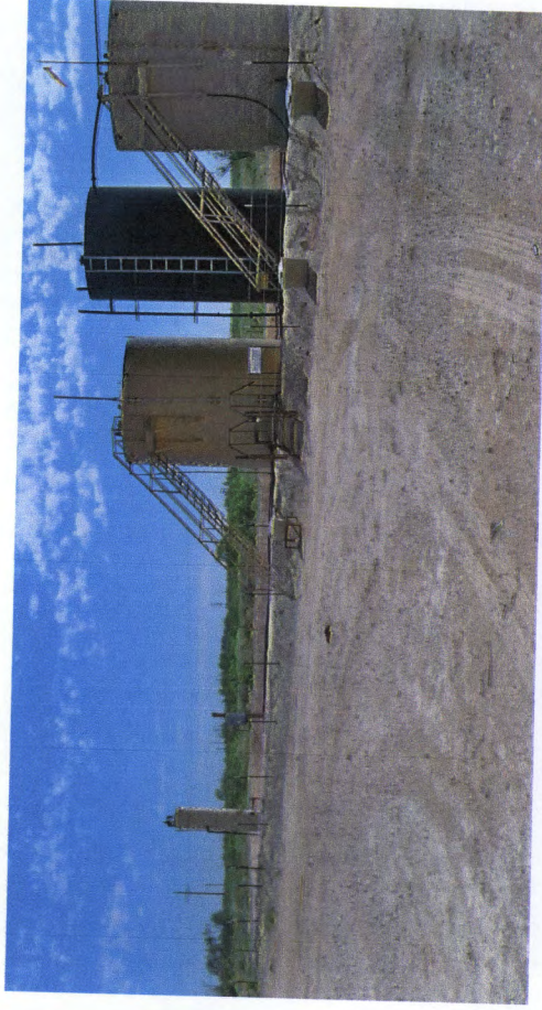
Water tank now inside battery berm with gun barrel and oil tank
