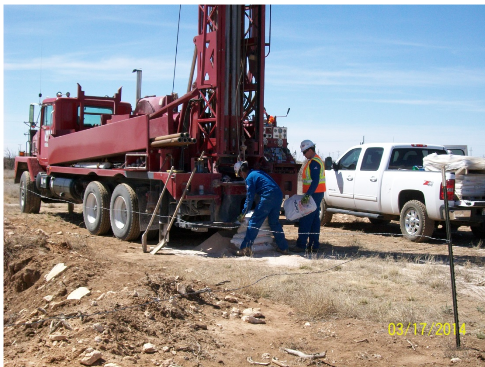
Photo 4 – View of 2014 boring backfill with bentonite pellets
