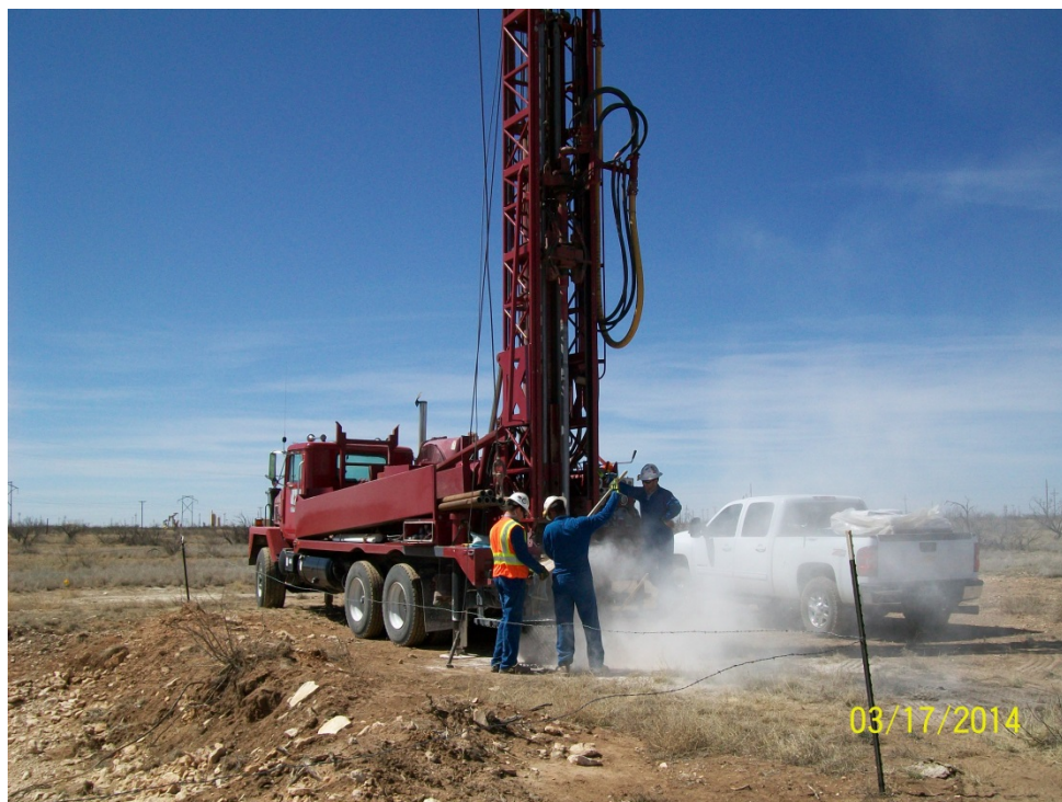
Photo 3 – View of 2014 soil boring advancement facing north west
