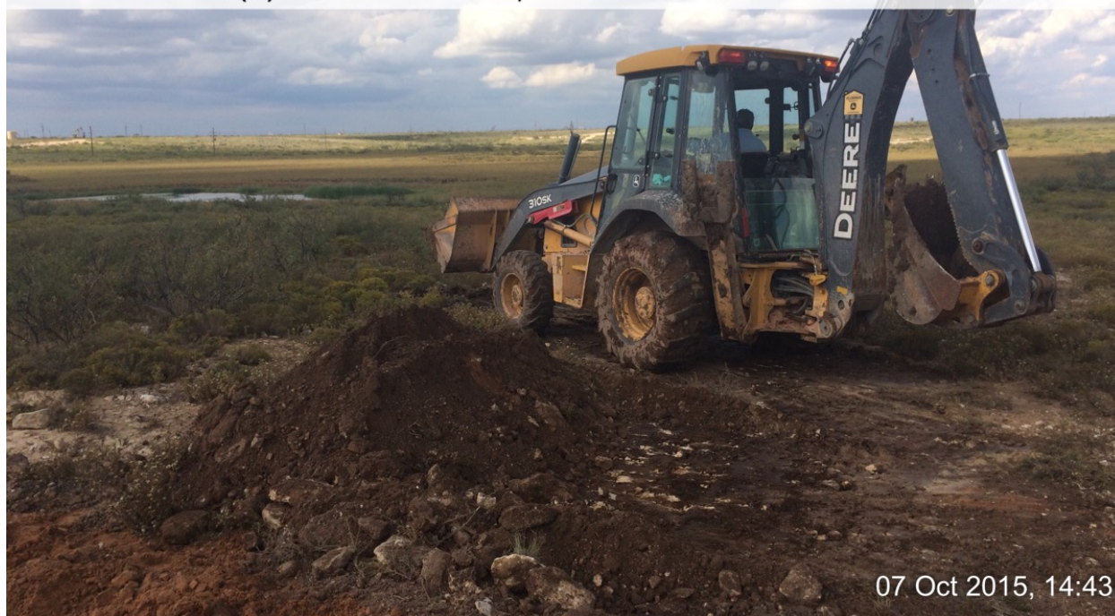
Initial scrape of the spill area
