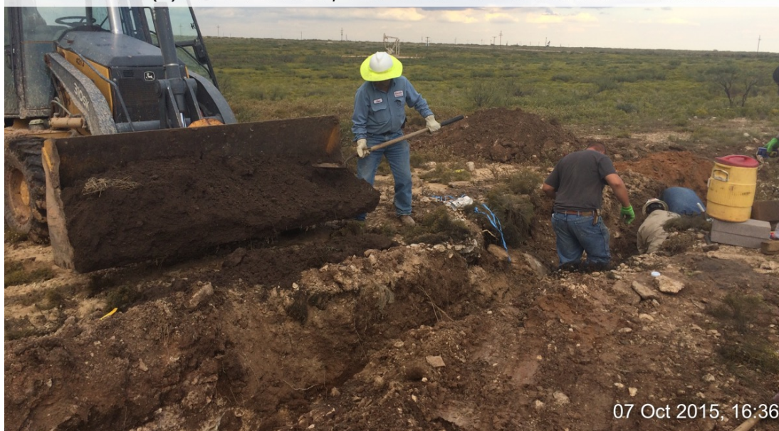
Digging out source of spill so crews could fix line
