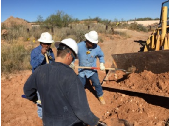
Hand digging/excavation around high pressure lines
