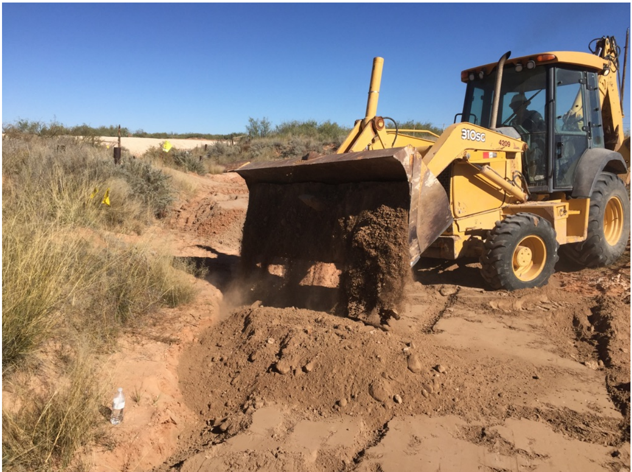
Excavating spill area
