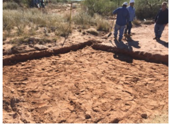
Hand digging/excavation around high pressure lines
