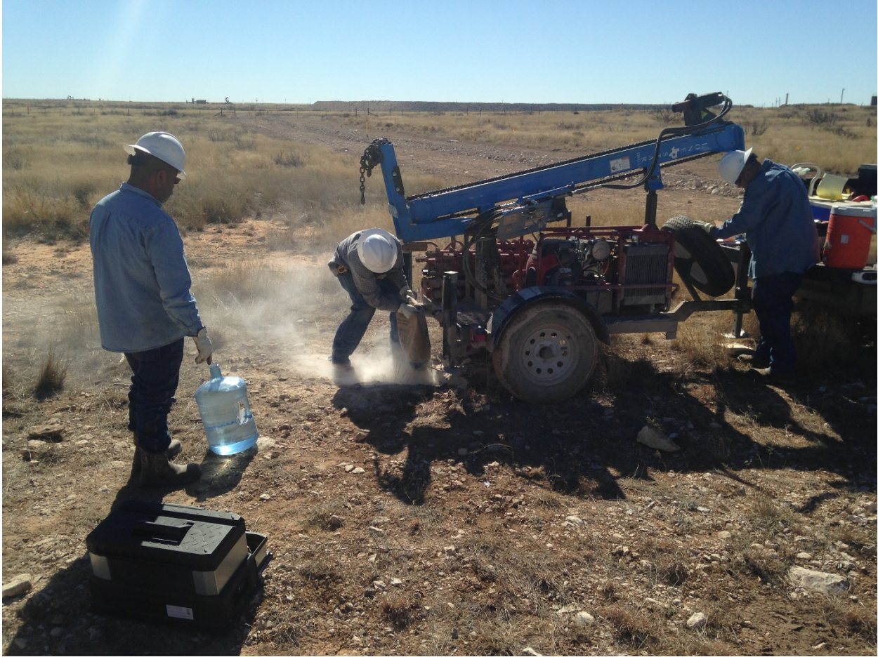
Plugging drilling hole with bentonite
