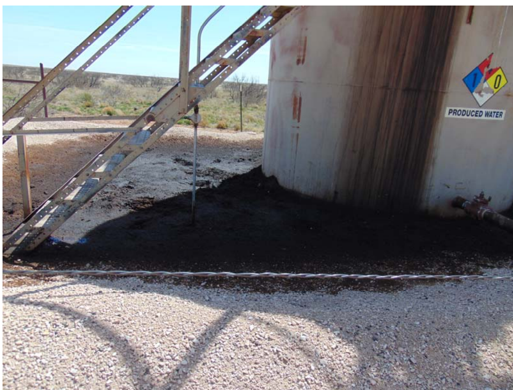
Photograph #2- Release with in containment berm.
