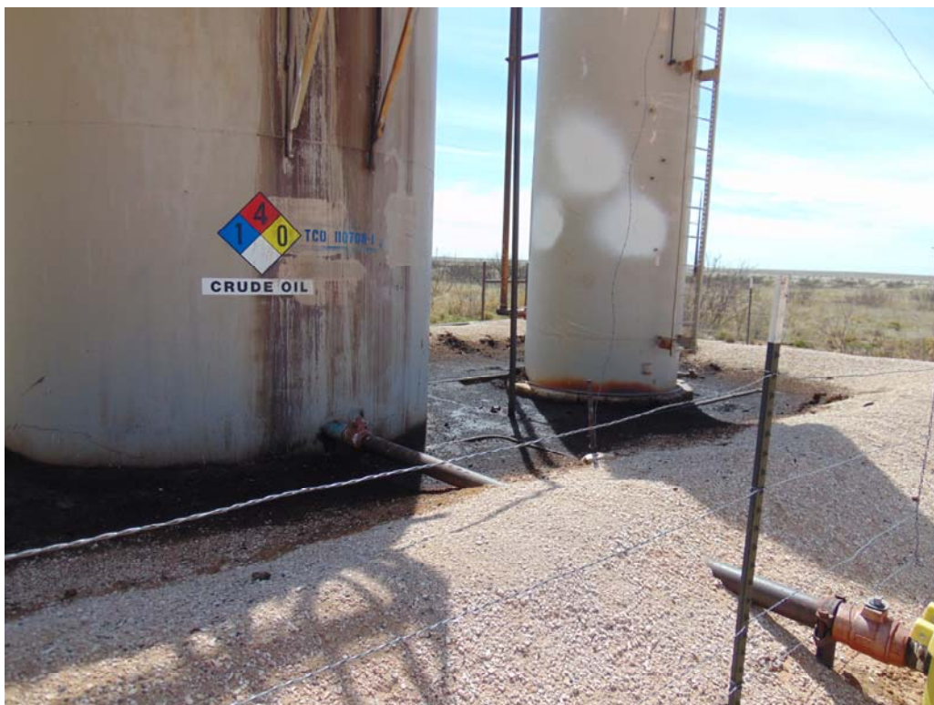
Photograph #4- Release with in containment berm.
