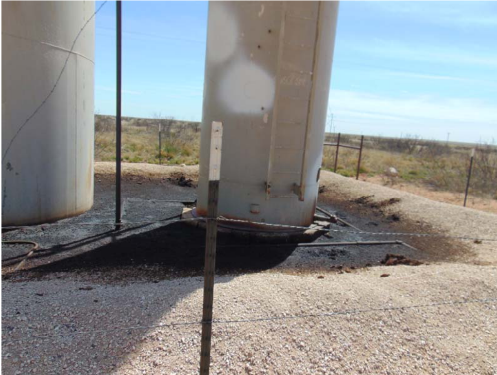
Photograph #5- Release with in containment berm.
