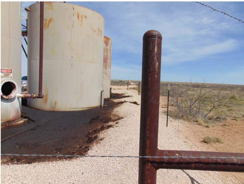
Photograph #6- Release with in containment berm.
