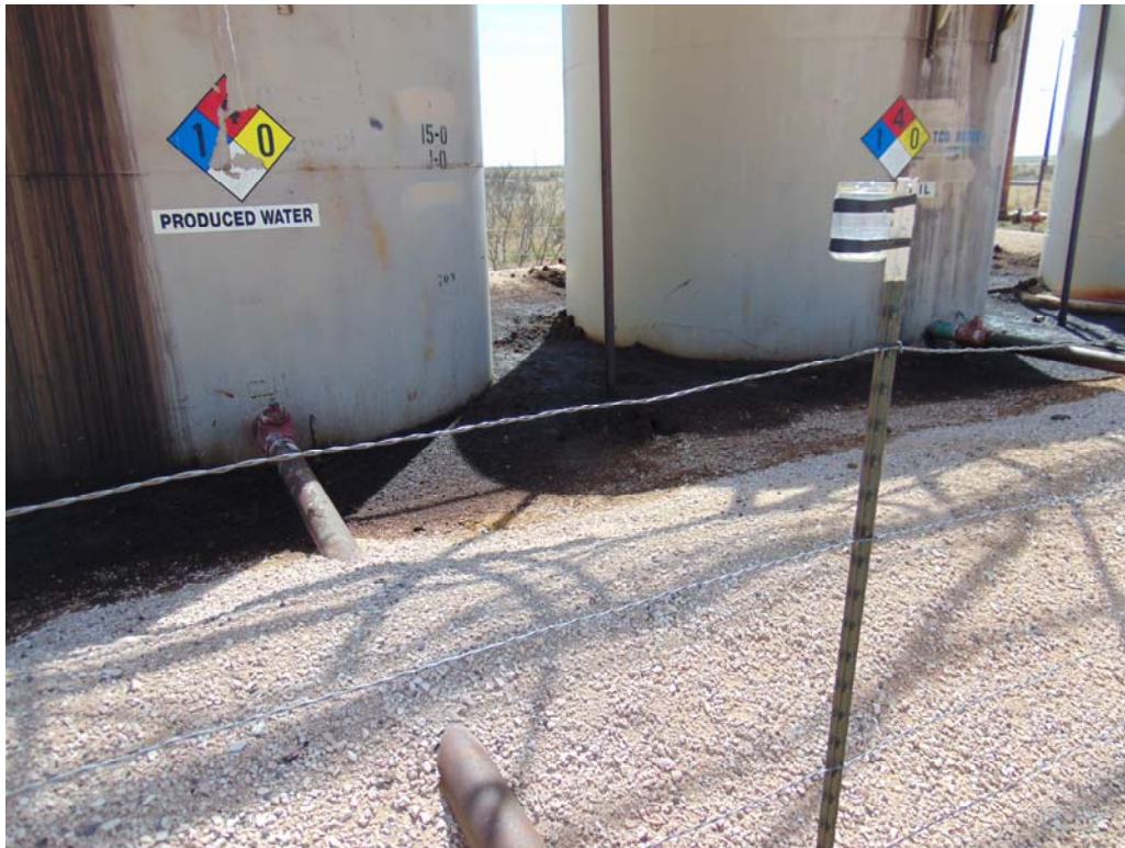
Photograph #3- Release with in containment berm.
