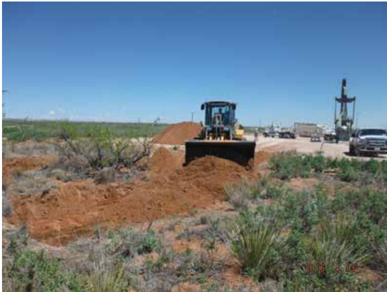
Backfilling Excavation, Facing North East 4/13/16
