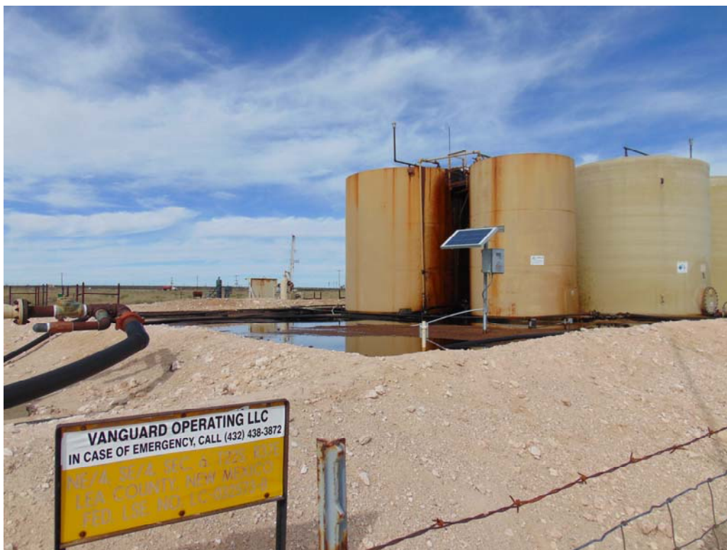
Photograph #1 – Release with in containment berm.
