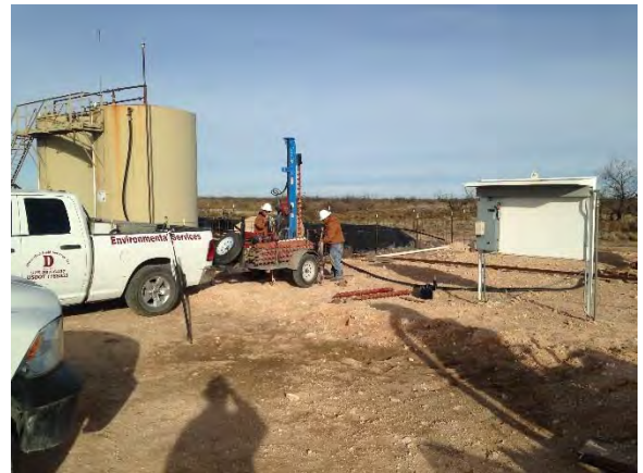
Installing soil bore, facing northwest
