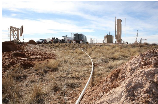
Leachate line to Frac Tank for recycling
