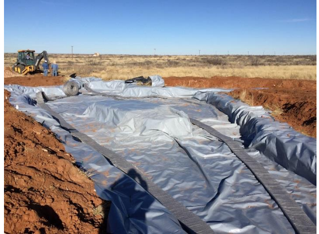
1-22-16 Liner Installation
