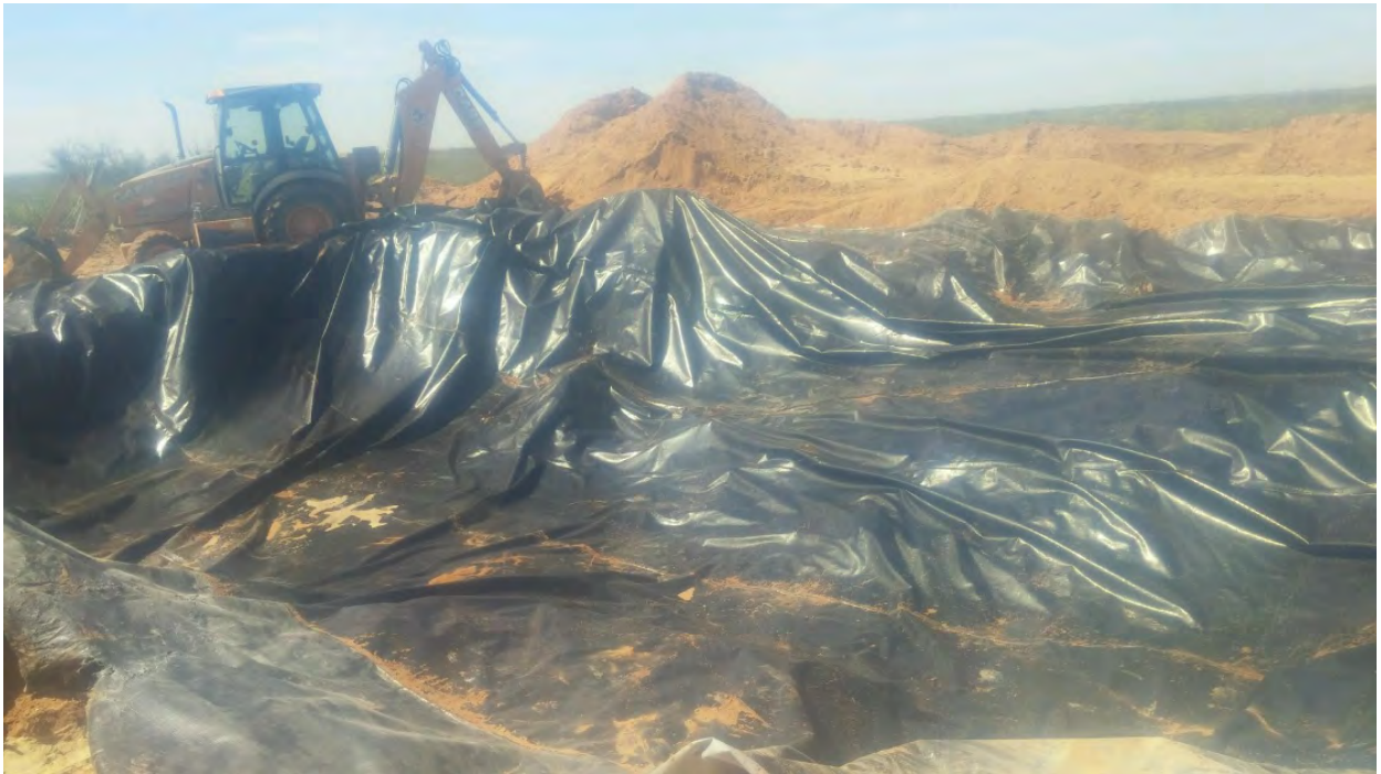
Photo 2 - Liner placement
