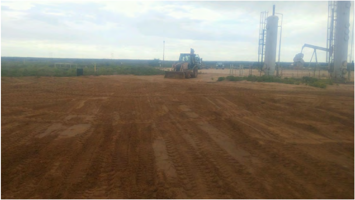
Photo 3 - Backfilled excavation, wheel compacted, re-seeded
