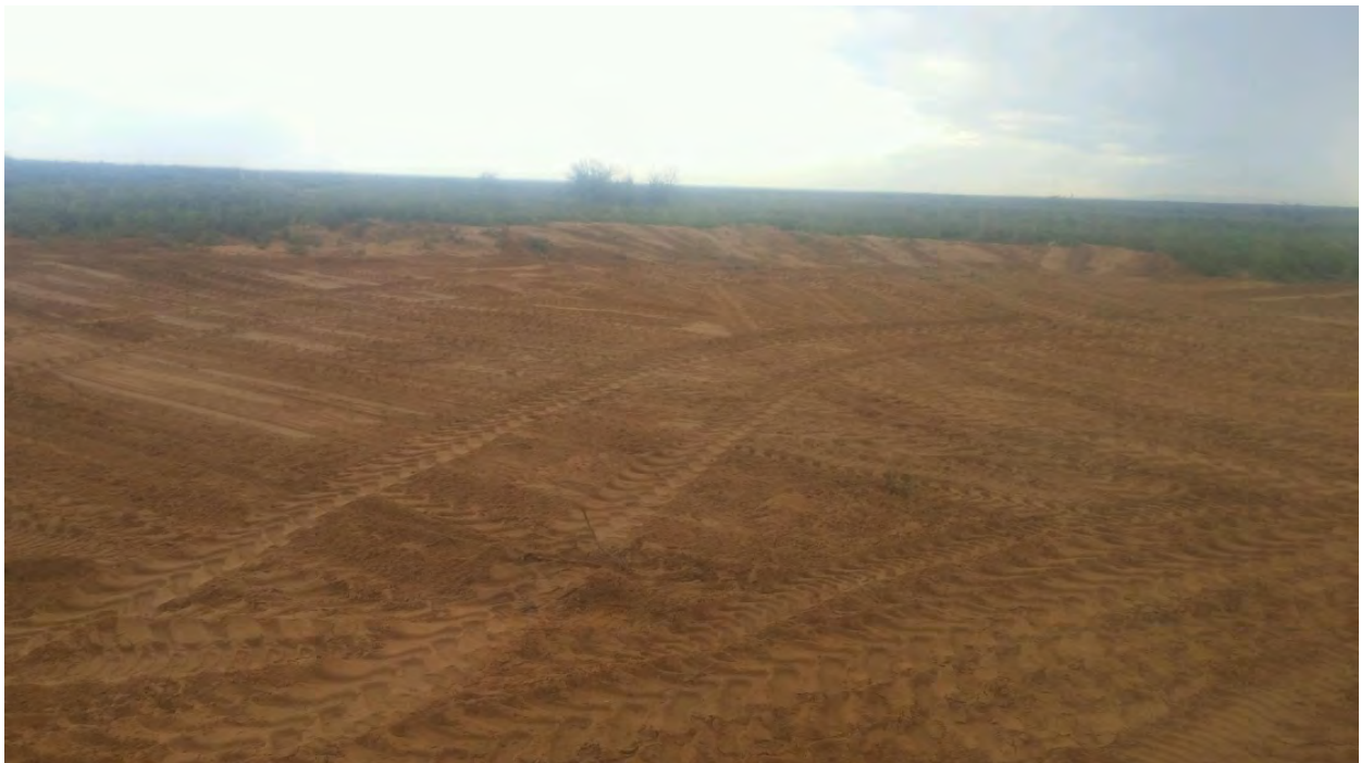
Photo 4 - Backfilled excavation, wheel compacted, re-seeded
