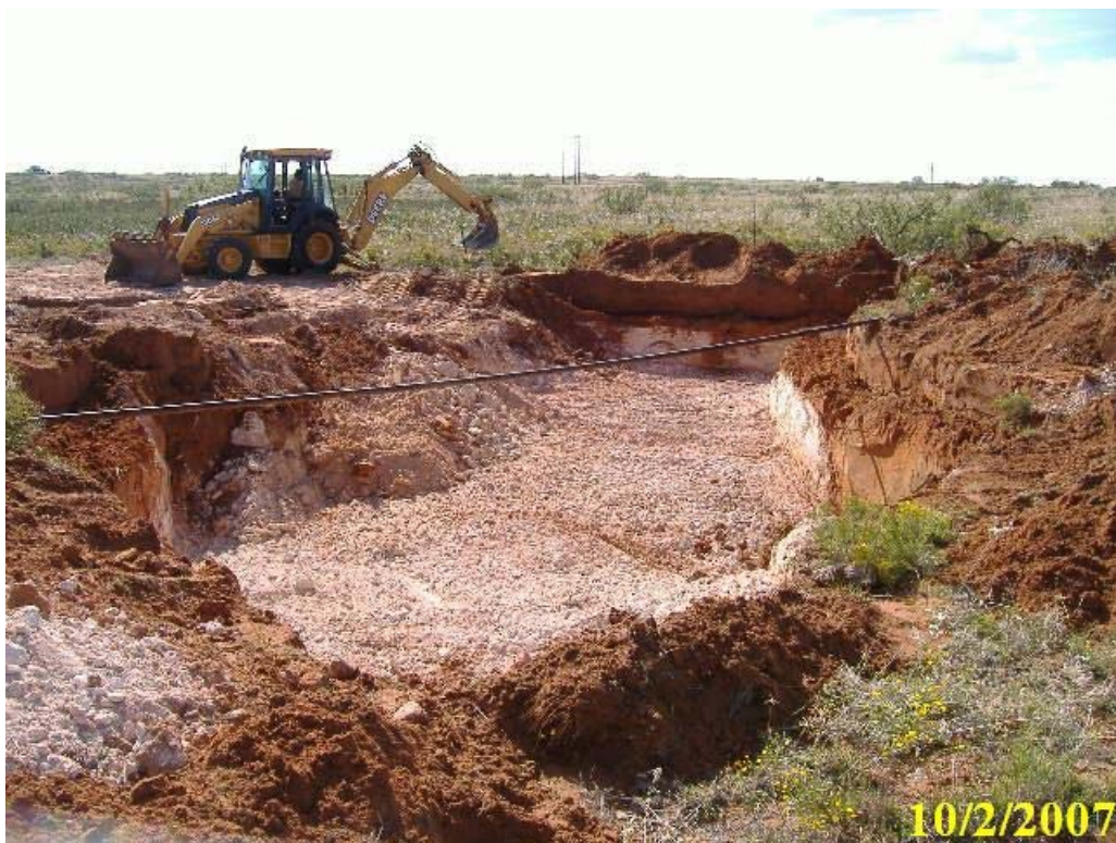
Photo #5 – Excavating contaminated soil
