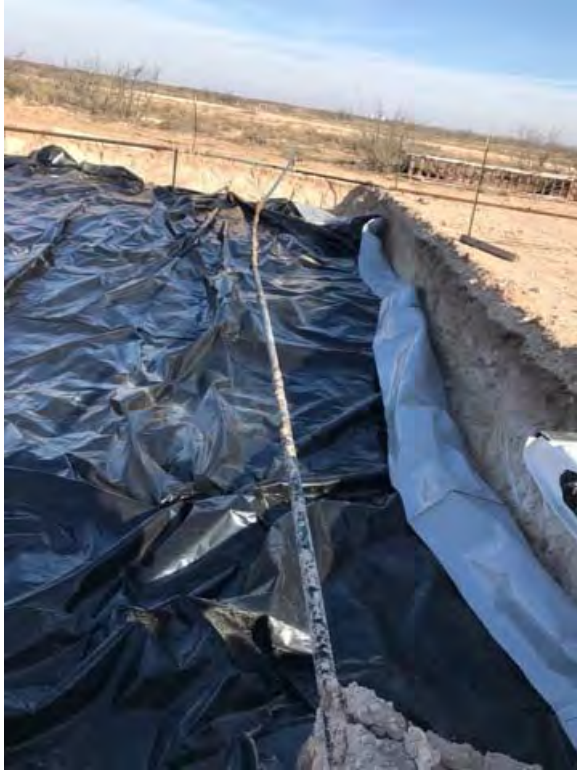
Installed liner at base of excavation
