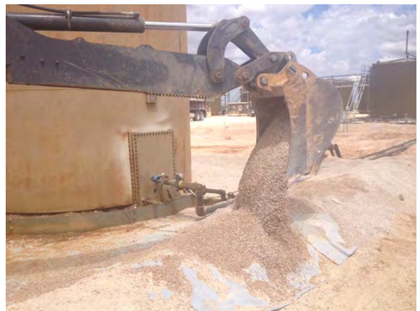
Backfilling site with caliche
