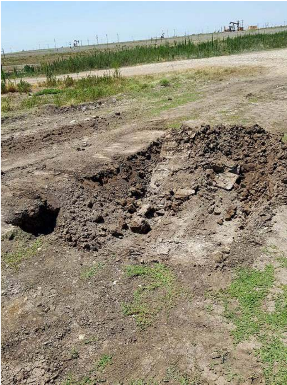
Facing NW: Additional excavating of impacted soil at DS-7 location on June 22, 2017. Confirmation sample was collected at bottom from 10-16"
