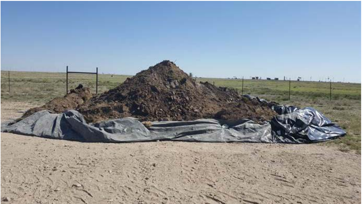
Facing South: Approximately 50 – 60 yards of impacted soil removed from release are
