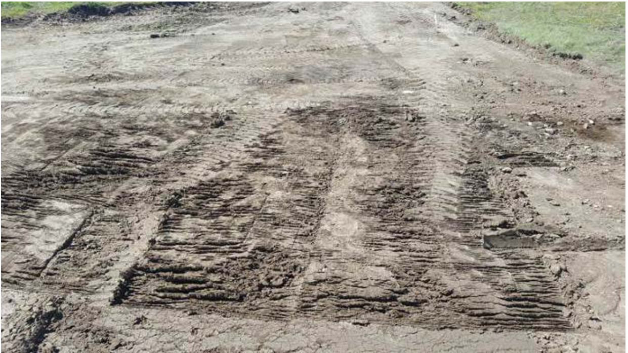
Facing North: Impacted soil scraped from release area
