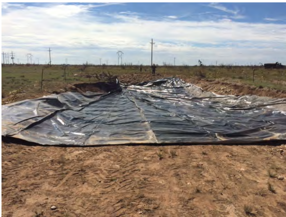
Photo 1 – View of liner placed within former excavation area.
