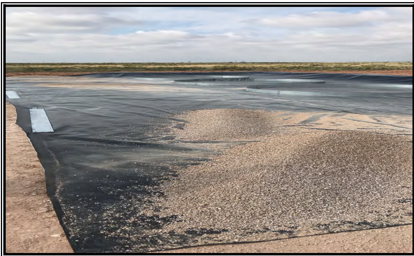
View of tank battery pad looking southwest after the installation of the plastic liner and tank ring bases.
