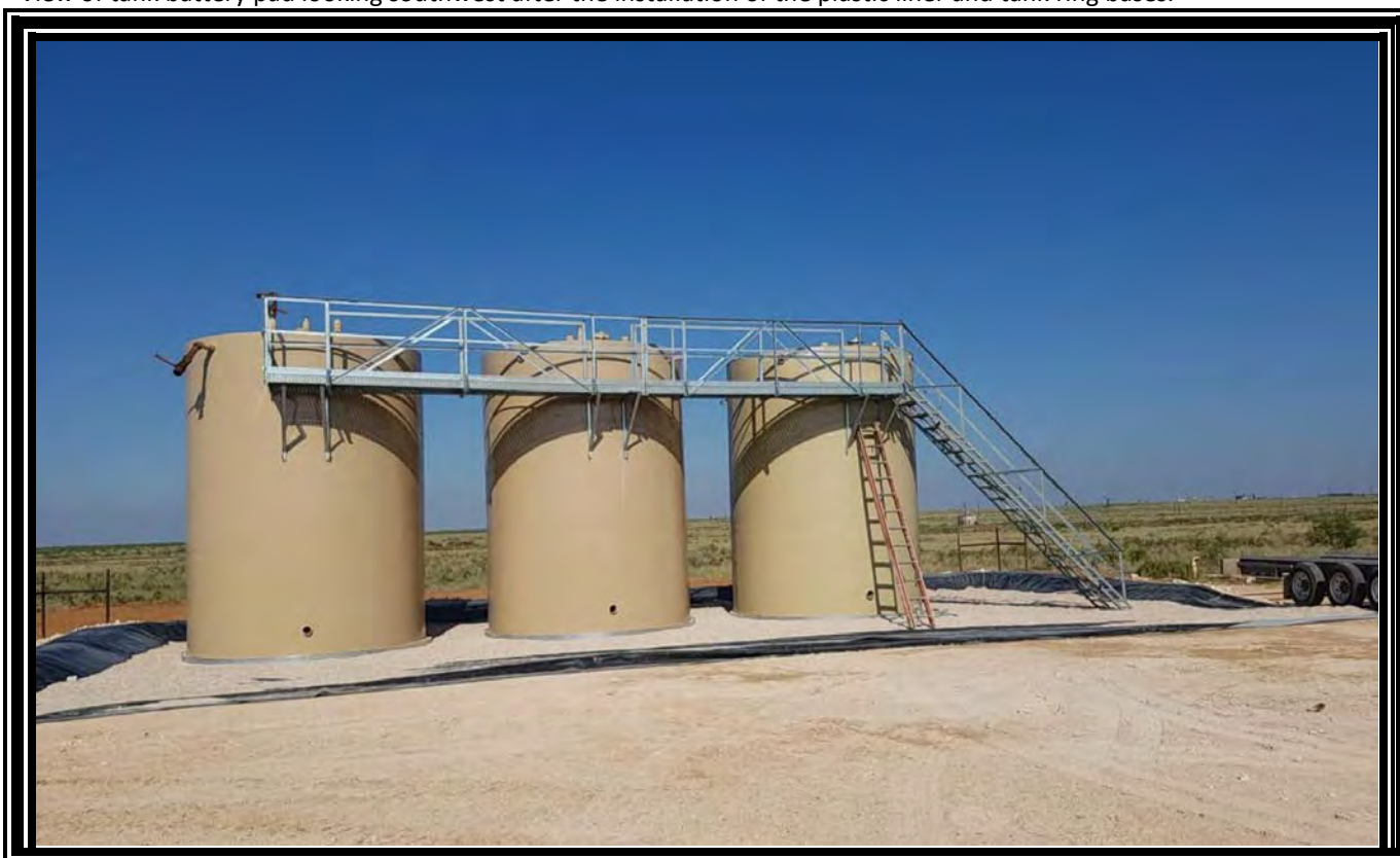
View of tank battery pad looking northwest after installation of tanks, stairs, catwalk, and pea gravel.
