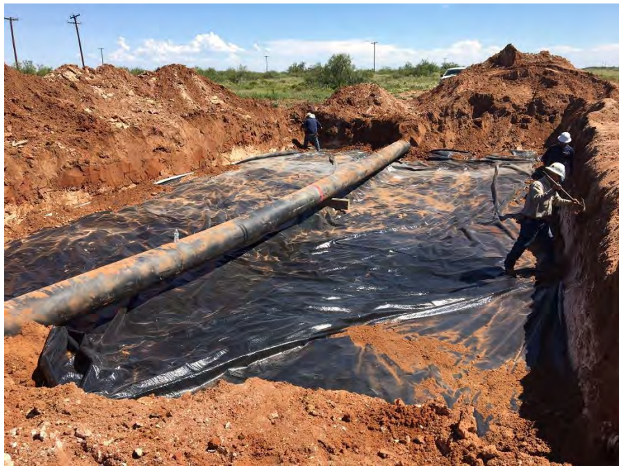
Photo 2 - Liner placement
