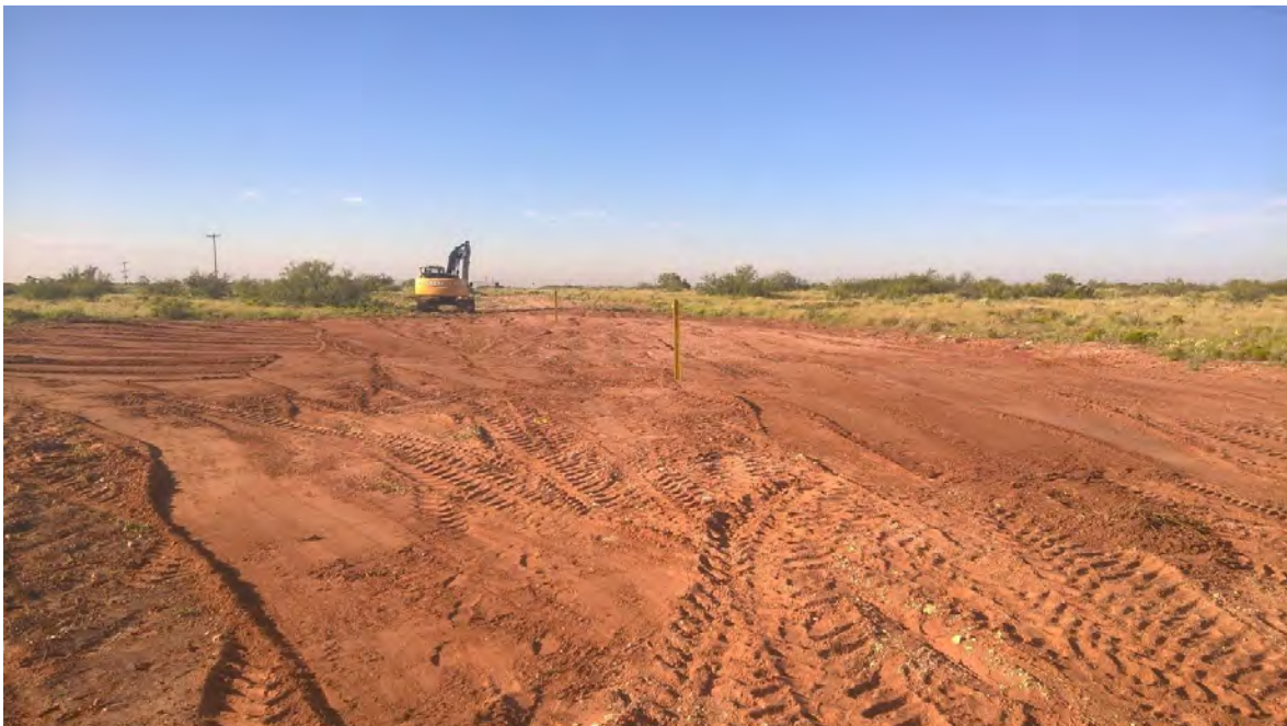
Photo 4 - Backfilled area
