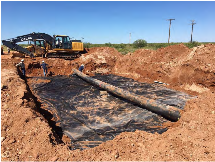
Photo 1 - Liner placement
