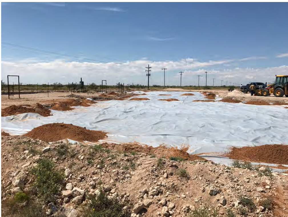
Merit 32 DM St. Com #1H – Liner Installation (Looking West)
