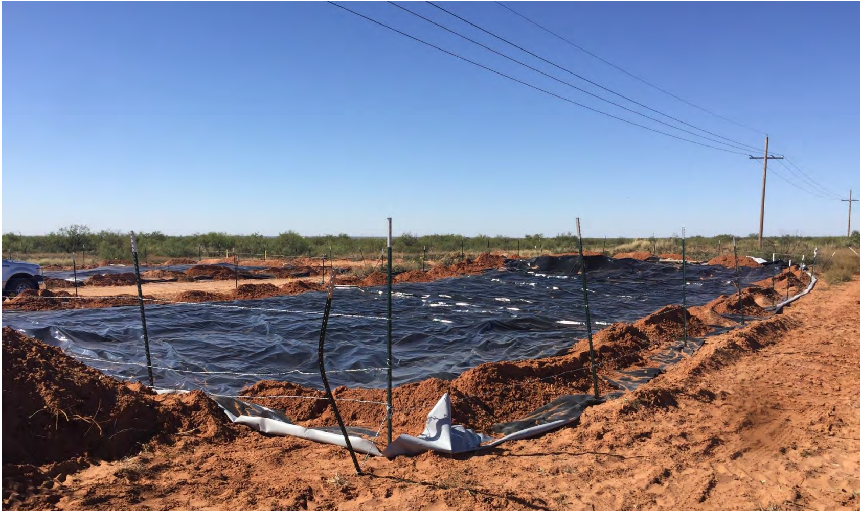
Photo No. 4. View of affected soil (north covered area) that was covered by 20 millimeter poly sheeting to prevent rainfall from causing further migration.
