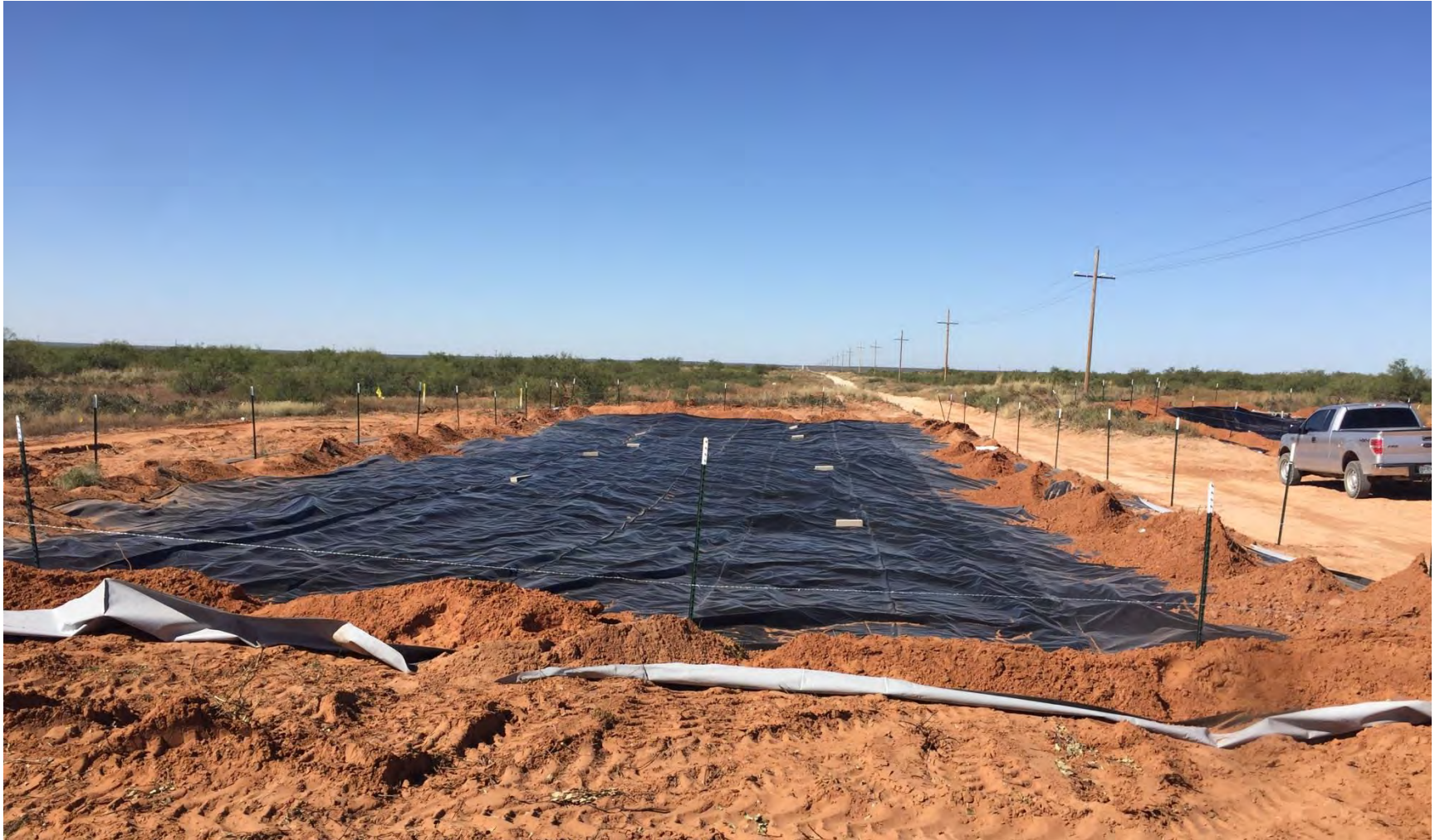
Photo No. 5. View of affected soil (south covered area) that was covered by 20 millimeter poly sheeting to prevent rainfall from causing further migration. NOTE: The NM811 identified multiple pipelines running parallel to the established caliche road.
