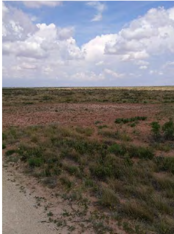
Photo 3 - Backfilled excavation, wheel compacted, re-seeded
