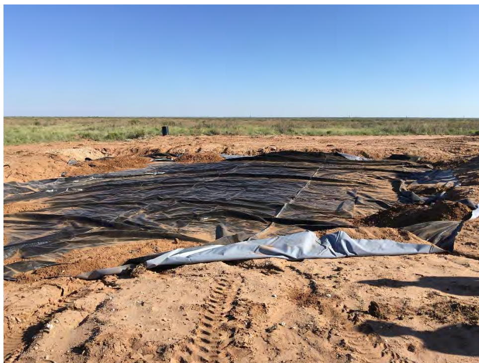
Photo 2 - Liner placement
