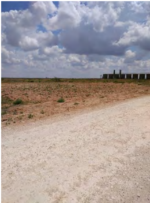
Photo 4 - Backfilled excavation, wheel compacted, re-seeded
