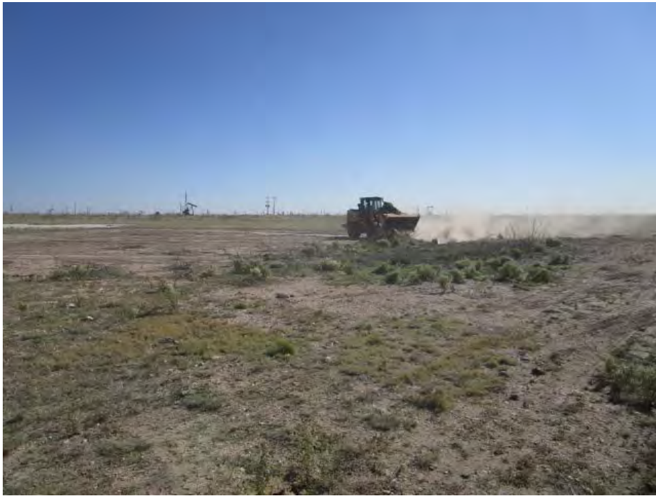
Photo 3 - Clearing, grubbing, and leveling the area to be lined
