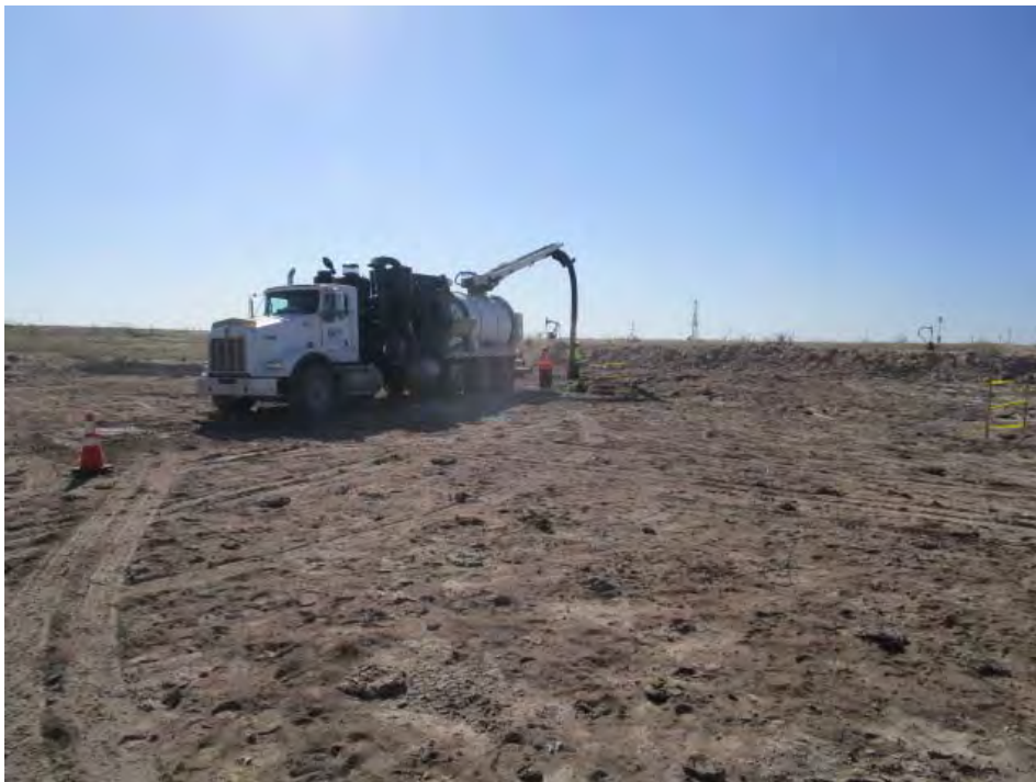
Photo 2 - Locating underground pipelines via hydrovac
