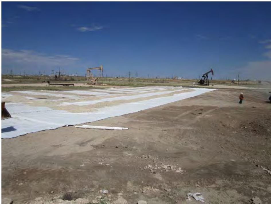
Photo 6 - Perforated pipe placed on top of underground pipelines and underneath the liner for leak detection
