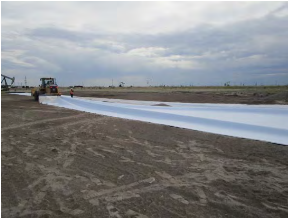
Photo 5 - Liner being placed
