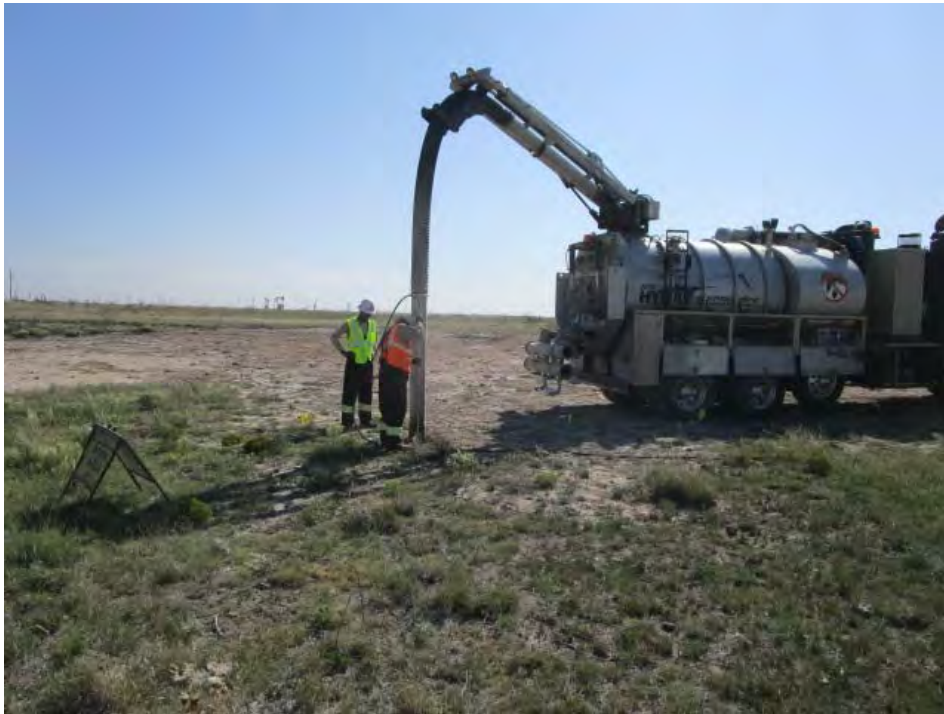
Photo 1 - Locating underground pipelines via hydrovac
