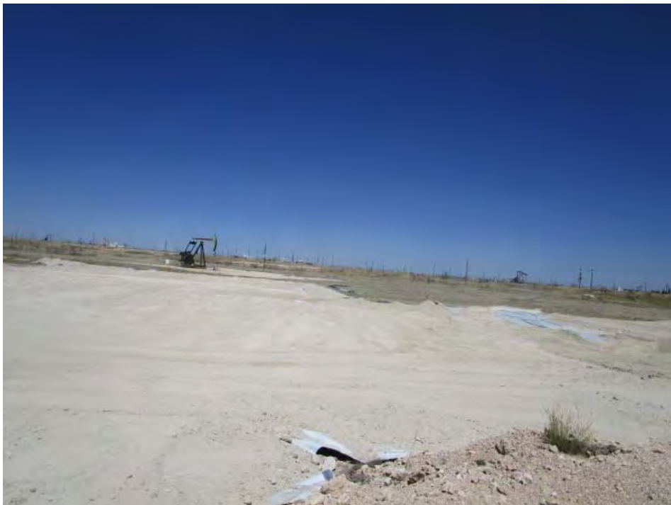
Photo 8 - Caliche placed on top of the liner to secure in place
