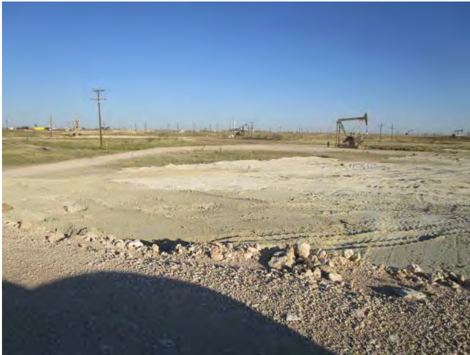
Photo 9 - Approximately one foot of caliche placement complete
