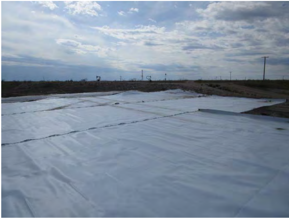
Photo 7 - Liner is placed over the entire cleared area
