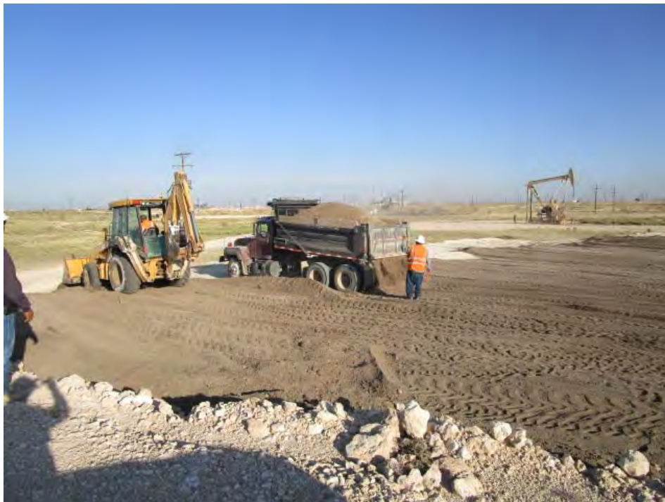
Photo 10 - Placement of topsoil on caliche
