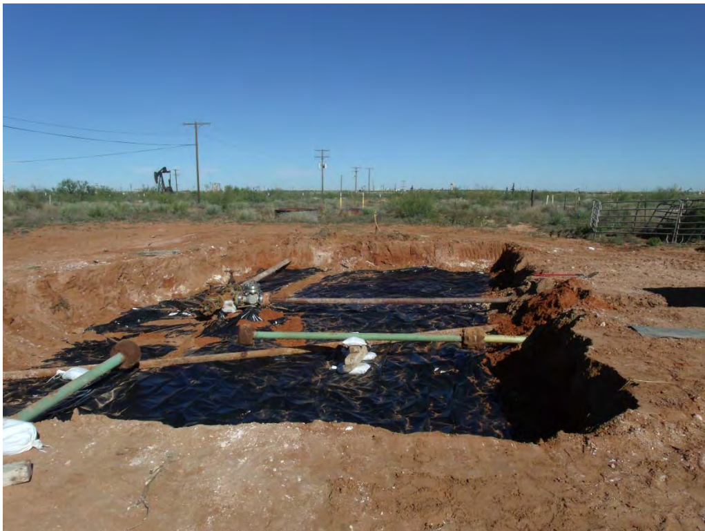
Photograph #10 – Liner installed
