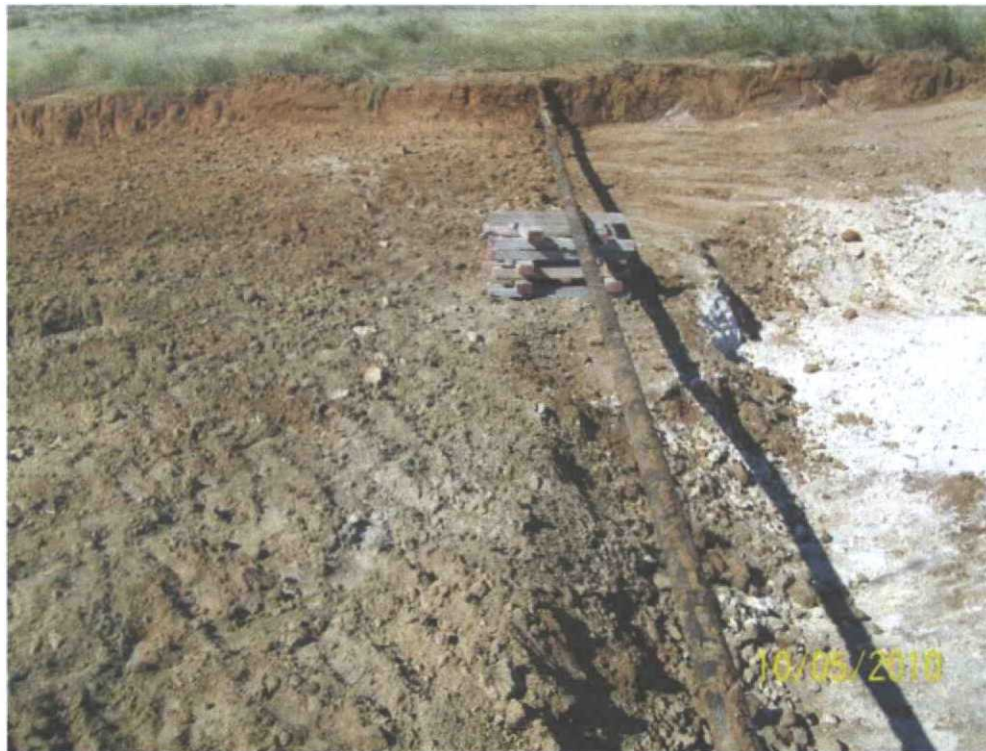
Photograph #4 – Looking northerly at initial excavated area and active pipeline supported with wooden brace
