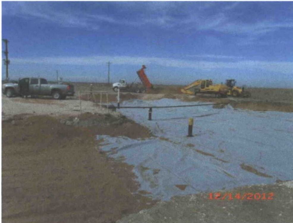
Photograph #9 – Looking north-westerly during liner installation.
